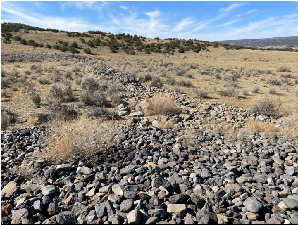
PL-21. Cutoff Wall Riprap
