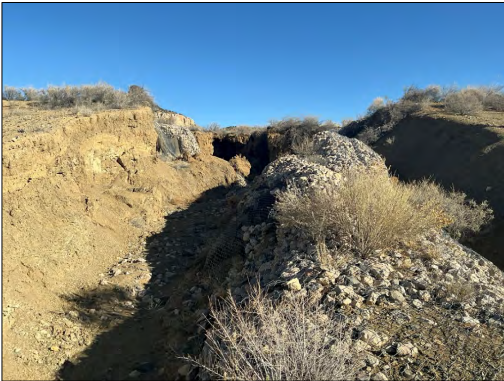
PL-18. Runoff Control Structure G
