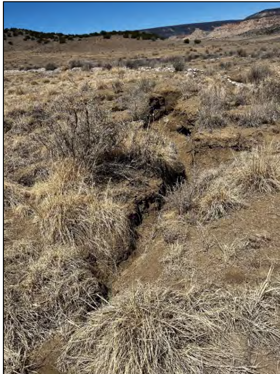
PL-19. Erosion near Runoff Control Structure A
