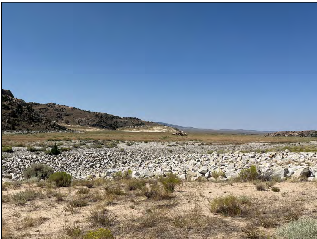
PL-18. Deep-Rooted Vegetation in Diversion Channel
