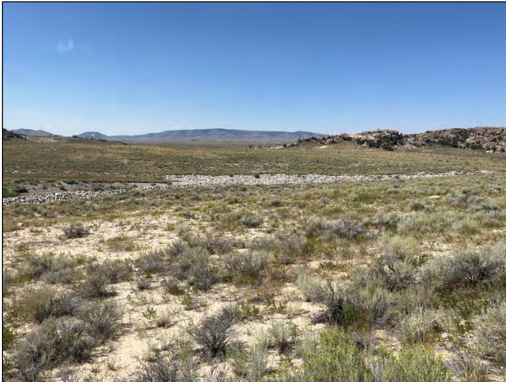
PL-11. Brush and Shrubs on Disposal Cell Side Slopes
