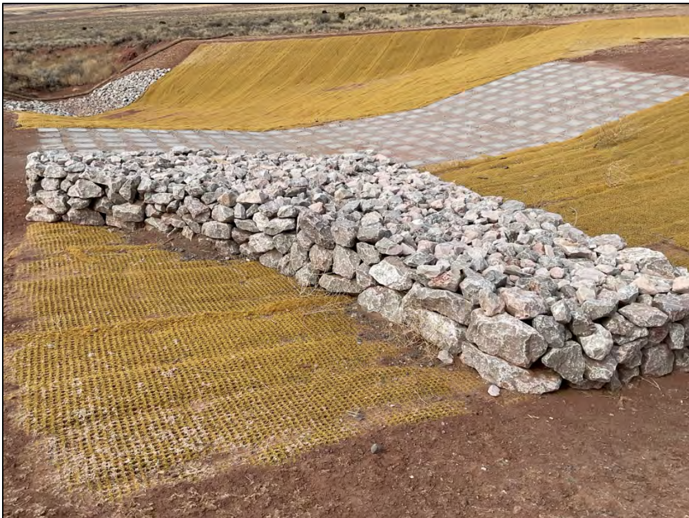
PL-2. Perimeter Access Road Low Water Crossing
