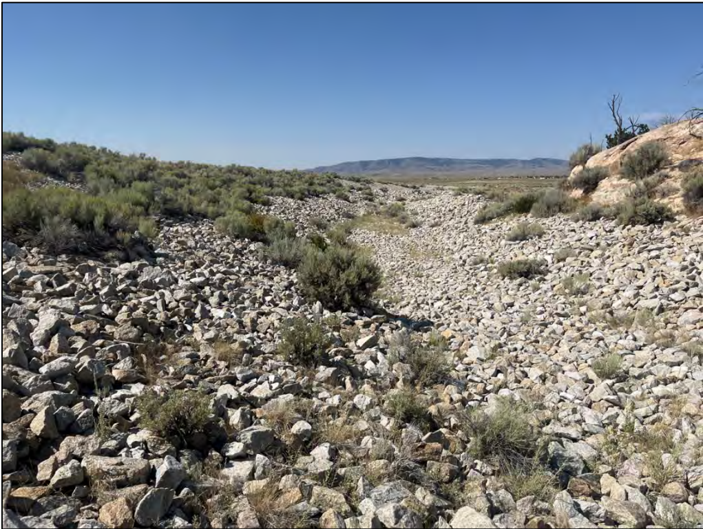
PL-16. South-Central Diversion Channel
