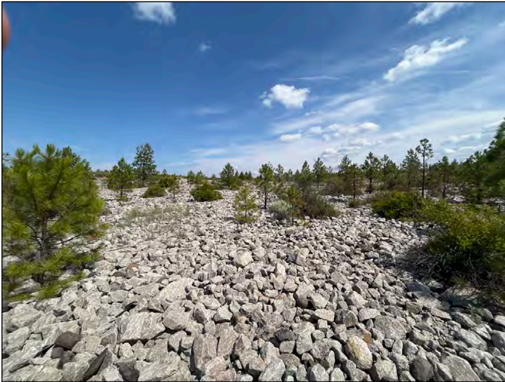
PL-5. Riprap-Armored Swale
