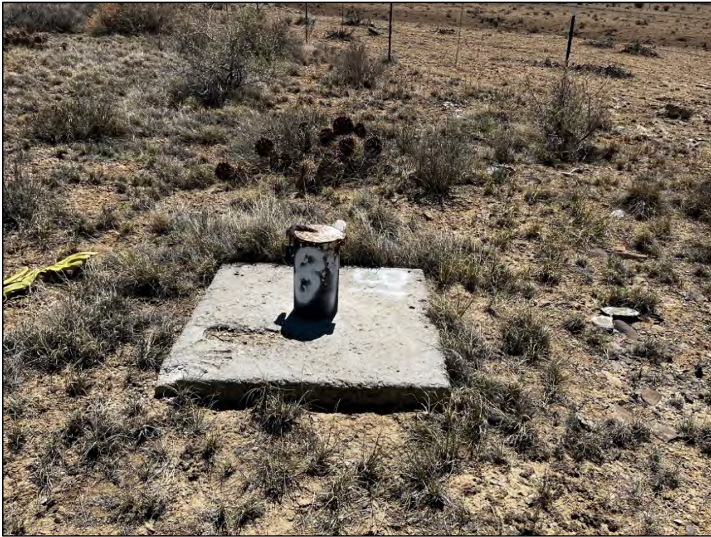
PL-13. New Paint at Monitoring Well 81
