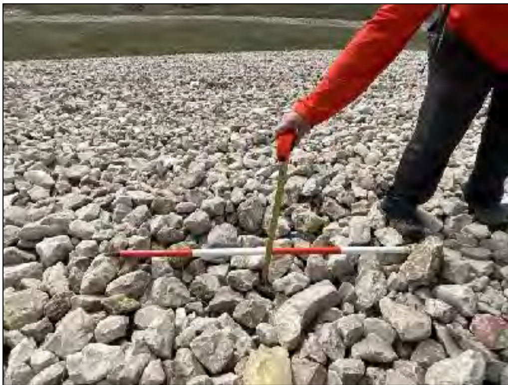
PL-3. Depression No. 2, Measuring Depth
