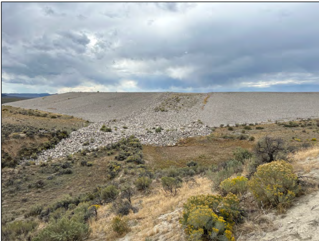
PL-10. Launch Rock Erosion Protection Basin
