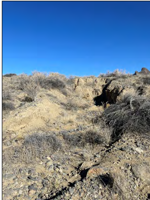
PL-8. Slope Erosion near Perimeter Sign P26
