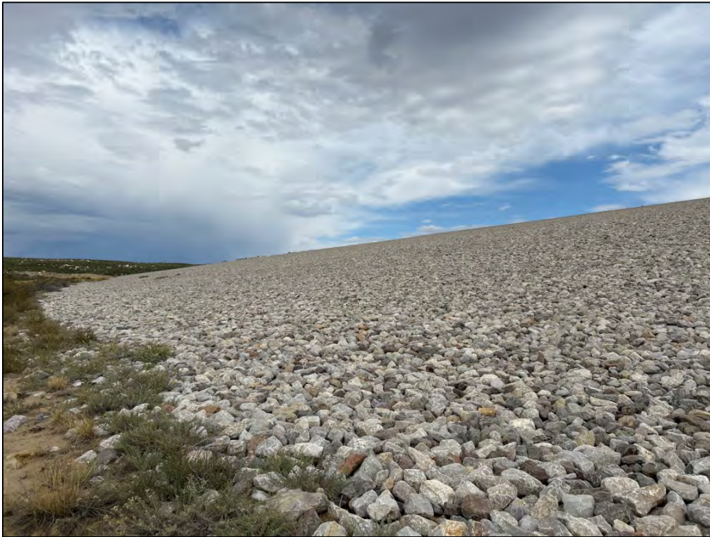
PL-7. West Side Slope of the Disposal Cell
