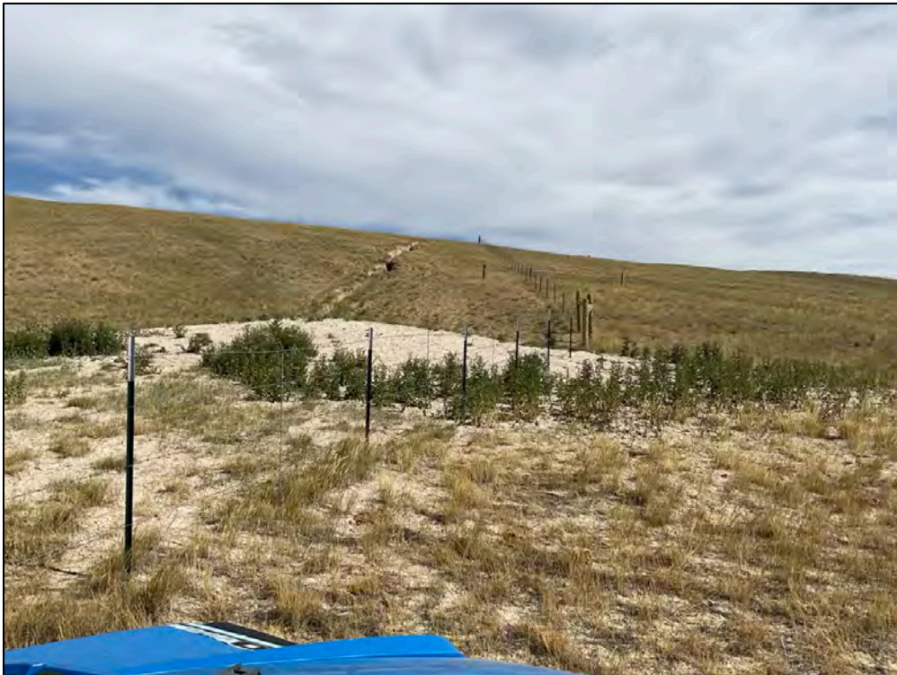
PL-2. Sediment Deposition Along Western Boundary
