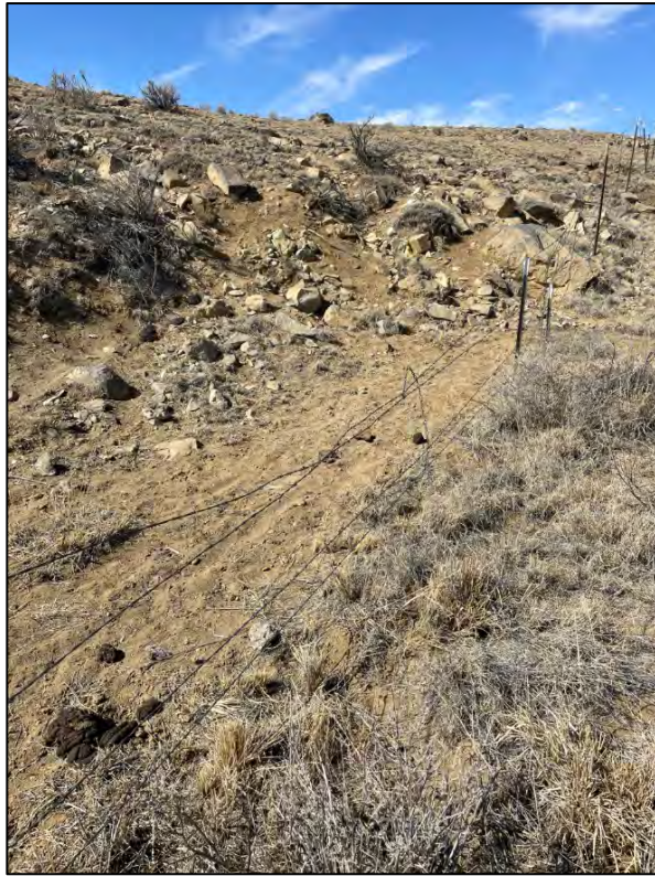
PL-5. Broken Fence
