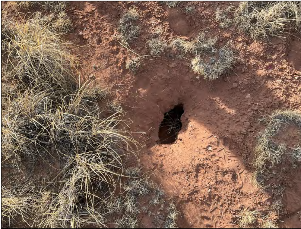
PL-19. East Dump Soil Piping
