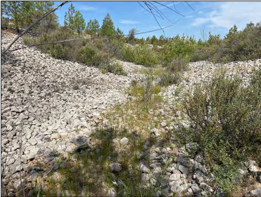
PL- 11. Riprap-Armored Diversion Channel
