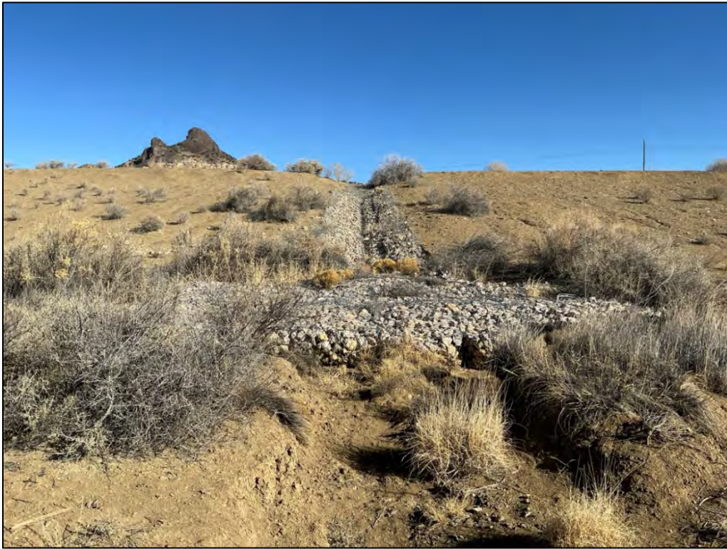
PL-17. Runoff Control Structure F
