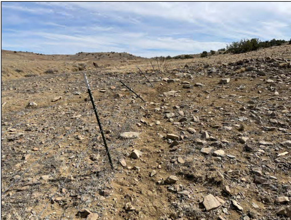
PL-6. Loose and Leaning Fence Line
