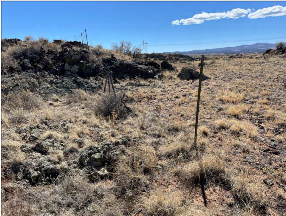
PL-3. Western Perimeter Fence Repair Section
