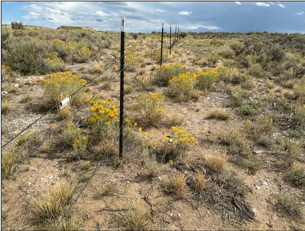
PL-1. Damaged Fence Line
