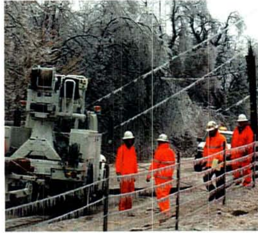
Linemen restoring electric lines after winter storm in Oklahoma
