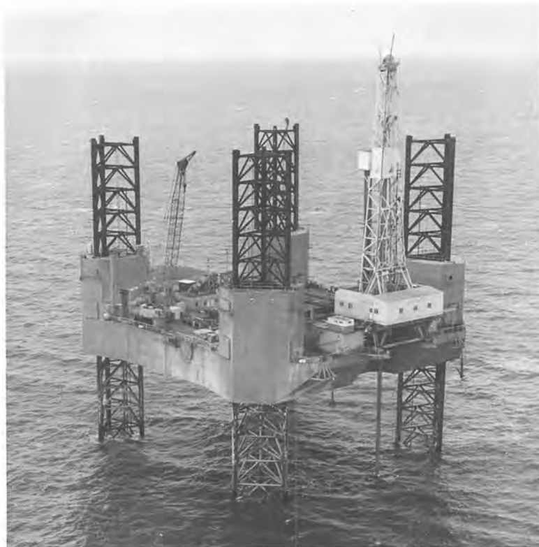
Figure 15. Fixed Platform Rig and Tender on Location.
