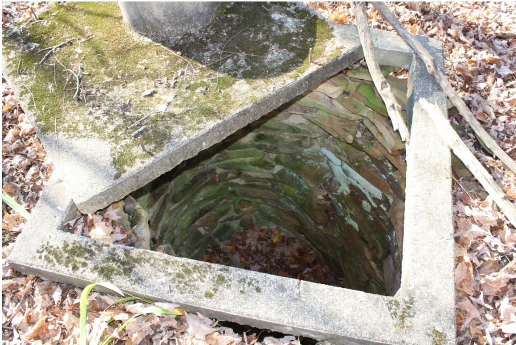
Figure 11. Photograph of cistern chamber (east).
