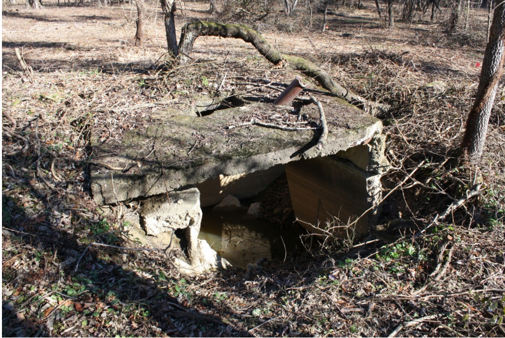
Figure 38. Photograph of the Mechling Farmstead cistern.
