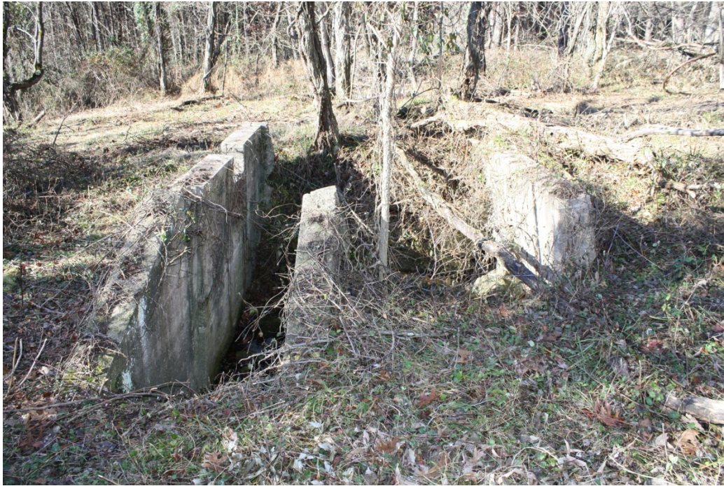
Figure 34. Photograph on the Mechling Farmstead House root cellar.
