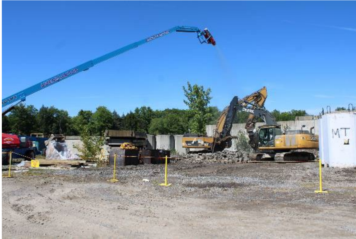
First VIT Vault to be demolished
