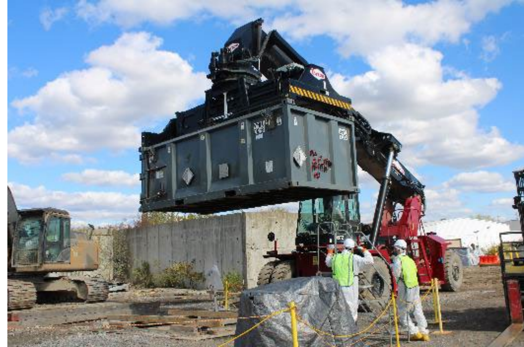
A reach-stacker removes a full waste container from the demolition area
