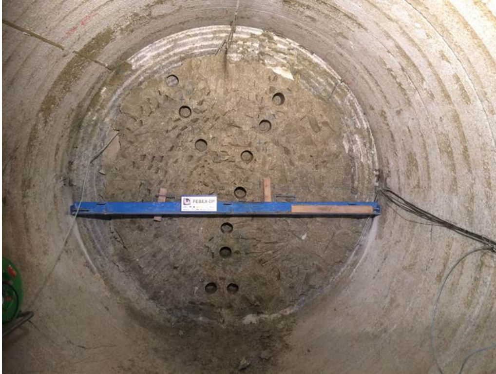
Figure 3-61. The front of dismantling section 62 with the core samples taken for microbiological studies, the blue bar prevents the partially detached bentonite from collapsing.
