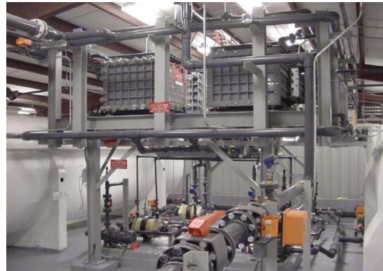
VRB (Prudent Energy) PacifiCorp (Moab, Utah) 2 MWh VRB-ESS
