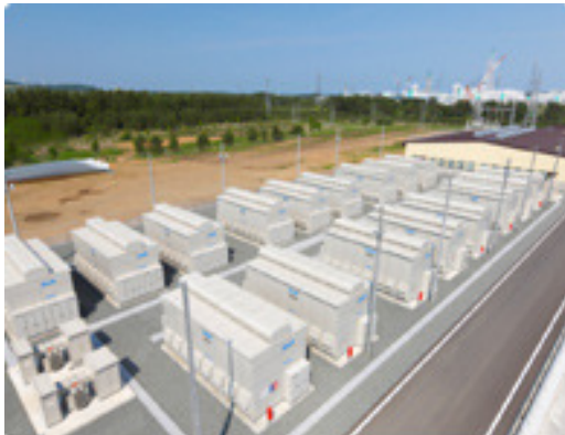
NGK 34 MW NAS alongside 51 MW Wind Farm
