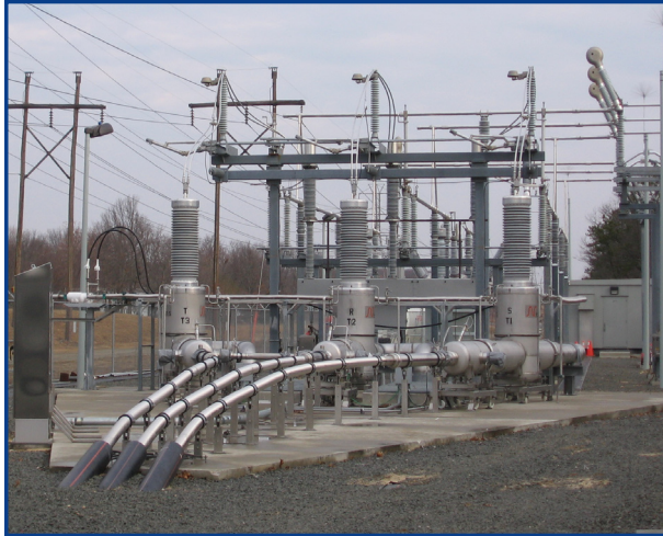
HTS cable at the LIPA substation.
