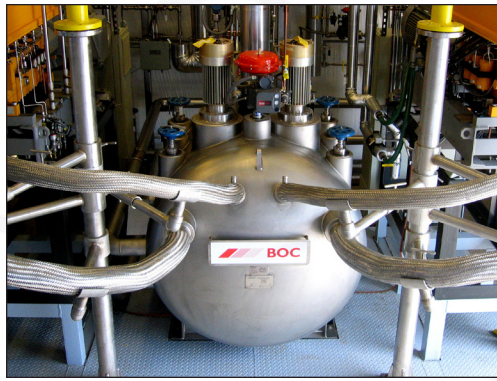
Linde's Cryogenic Refrigeration System (CRS)
