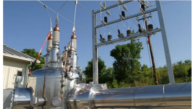
Albany HTS Cable Project — cable termination
