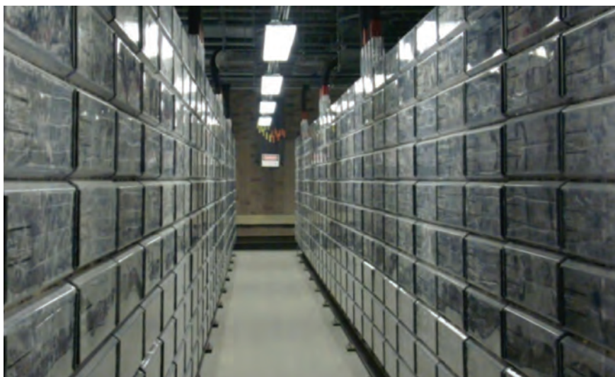
LEAD-CARBON BATTERY STACKS AT EAST PENN MANUFACTURING PLANT; DOE FUNDING FROM THE AMERICAN RECOVERY AND REINVESTMENT ACT
