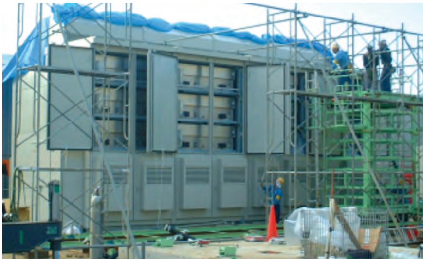
34-MEGAWATT, 7-HOUR SODIUM-SULFUR BATTERY ROKKASHO, JAPAN
