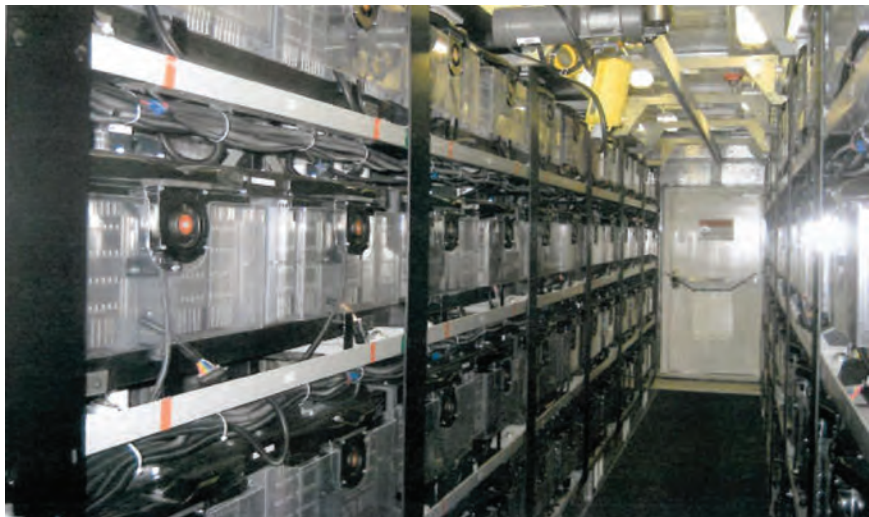
4 X 1-MEGAWATT, 15-MINUTE LITHIUM ION SYSTEM IN PJM INTERCONNECTION
