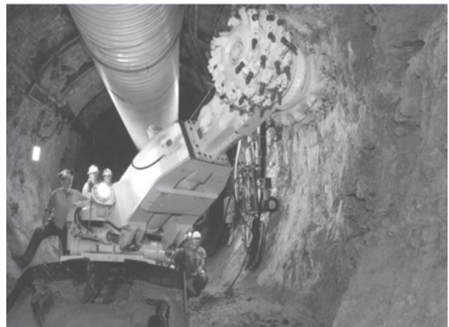
An "alpine miner" excavates an access tunnel inside Yucca Mountain. The Office of Civilian Radioactive Waste Management continues to conduct site characterization studies of the Yucca Mountain Site.
