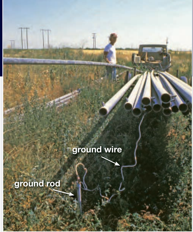
The possibility of nuisance shocks can be eliminated by grounding metal pipe when unloading near BPA lines.
