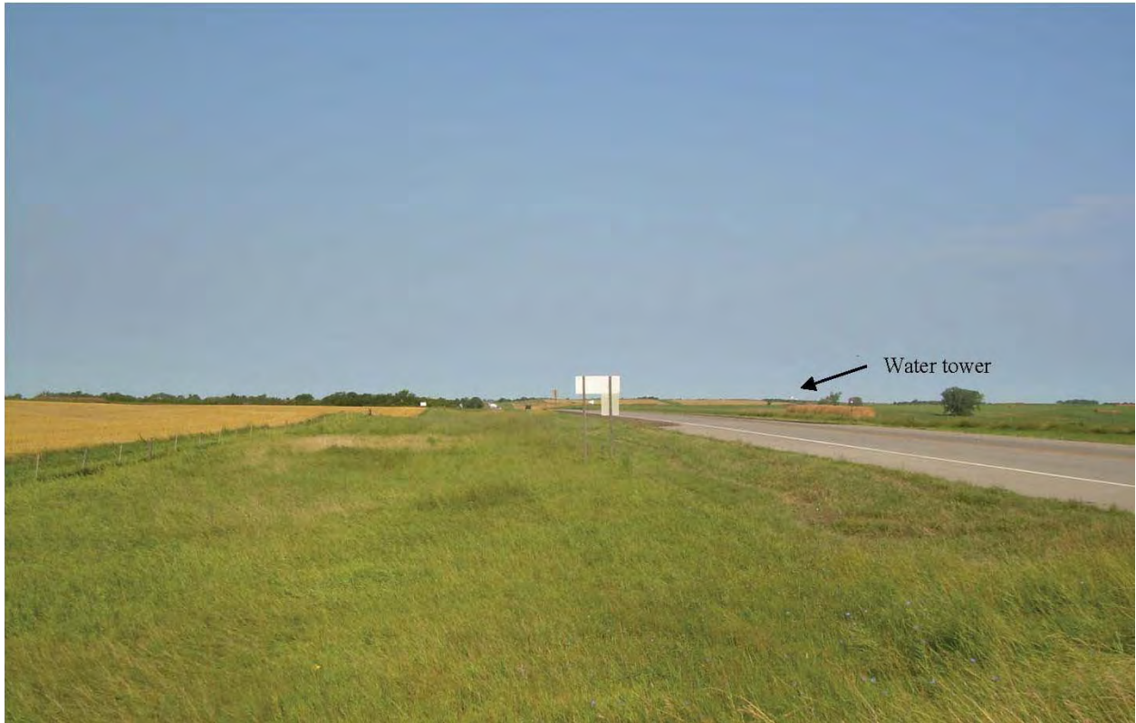
Figure 3.8-8 KOP 7 Existing Condition
