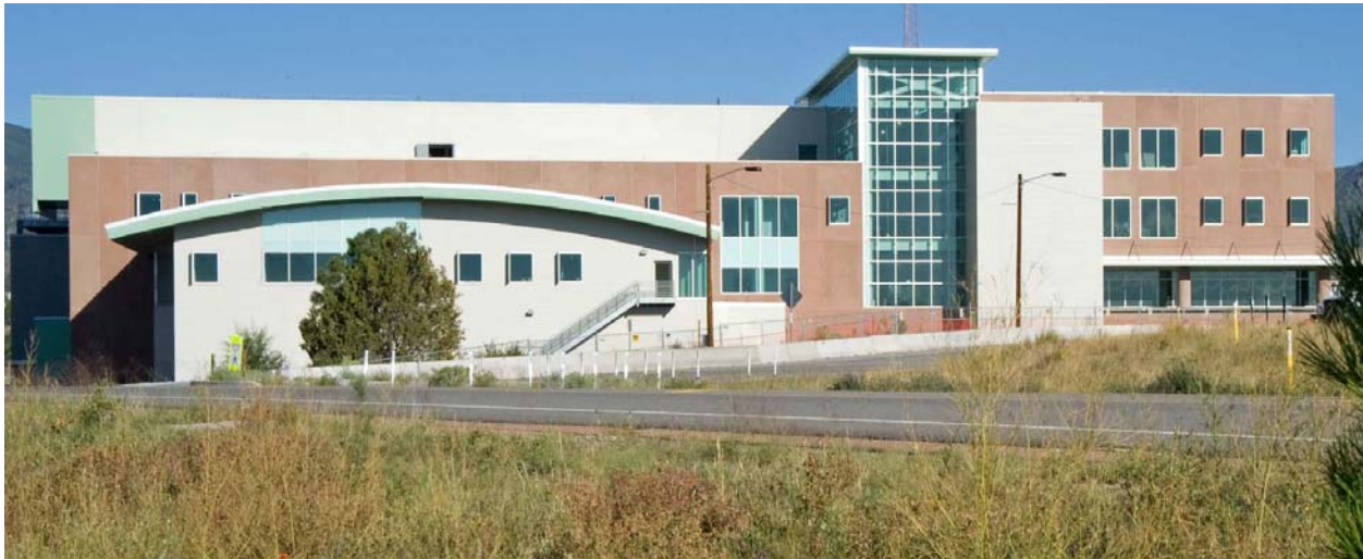
Figure 2–3 Radiological Laboratory/Utility/Office Building in Technical Area 55
