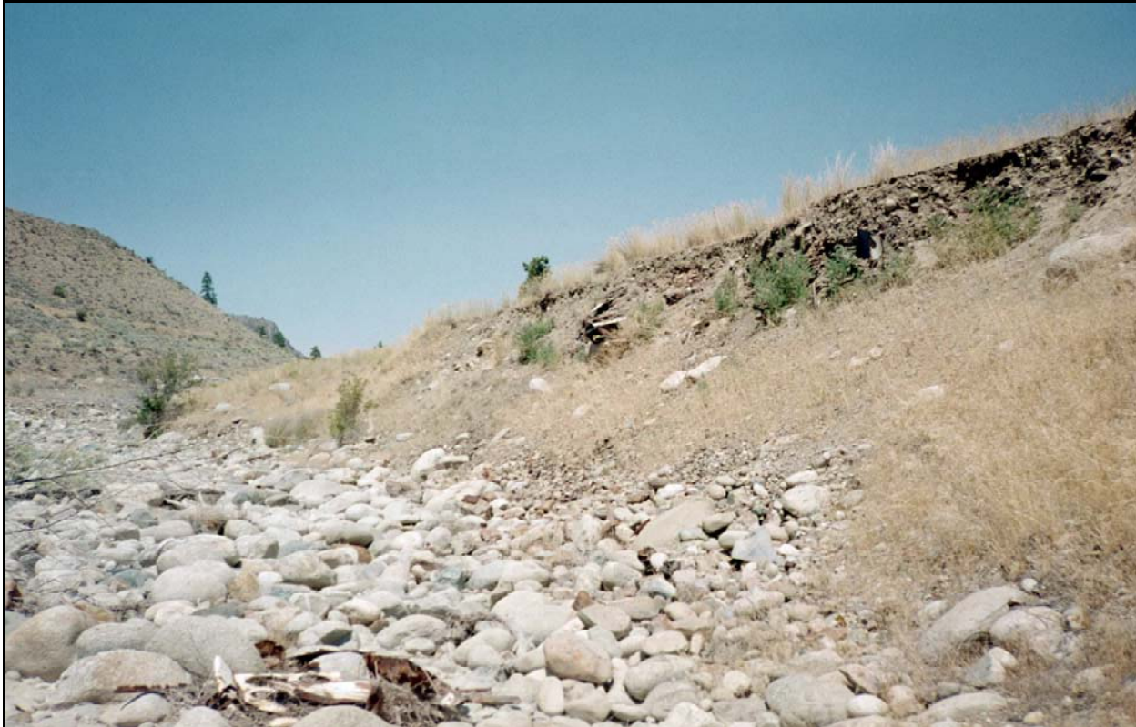
Figure 3-25. Salmon Creek Streambank with Debris Visible in Top Third of Bank. Note Lack of Streambank Vegetation and Water in the Stream Channel.
