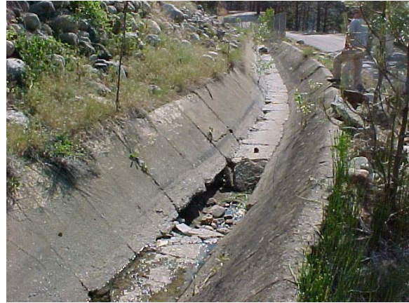
Figure 2-2 Existing Salmon Lake Feeder Canal
