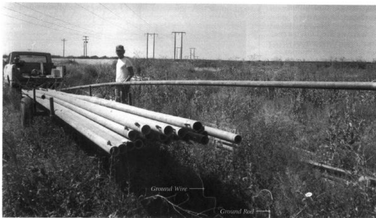
The possibility of nuisance shocks can be eliminated by grounding metal pipe when unloading near BPA lines.
