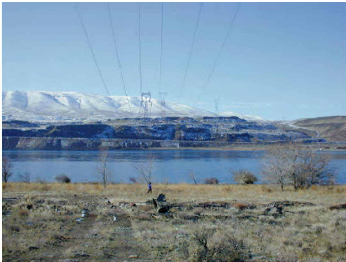
Photo 4.8-3. Visual simulation of Segment B looking west across the Columbia River near the Vantage Substation (General View 2 — See Photo 3.9-7 for original photo)
