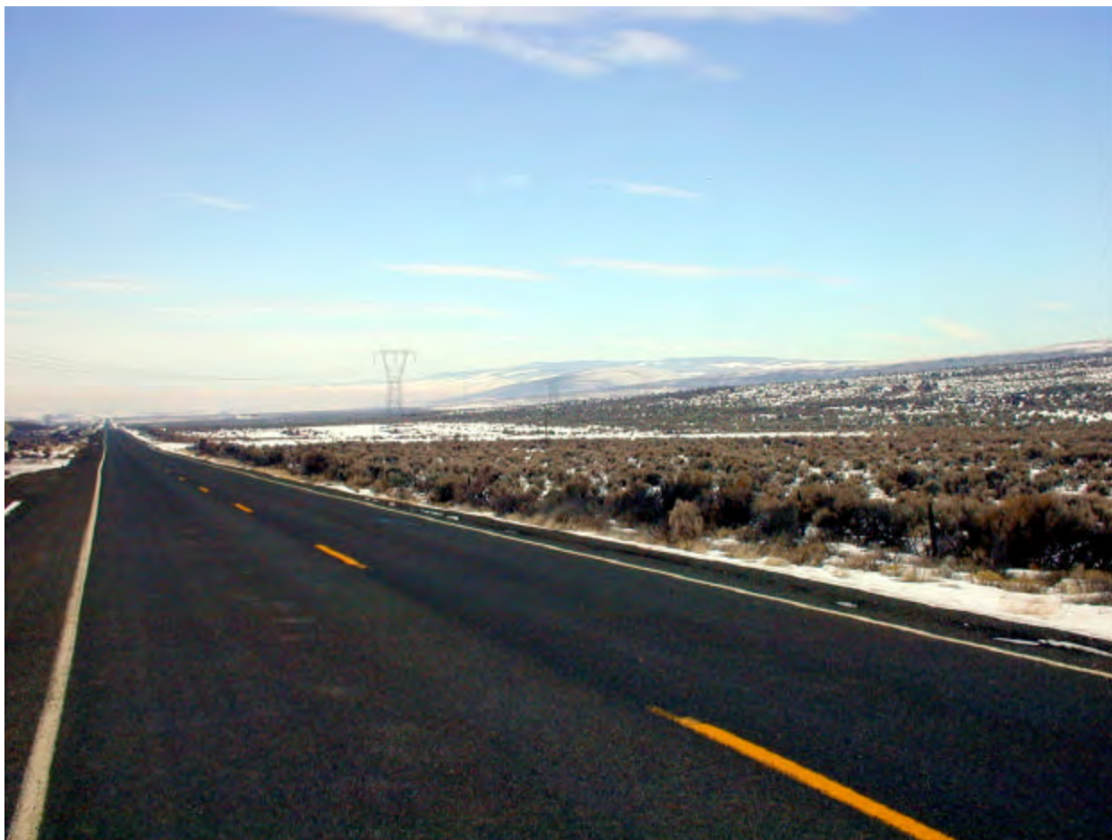
Photo 3.9-5. View of Schultz-Vantage transmission line crossing of Vantage Highway (View 1 on Map 10)
