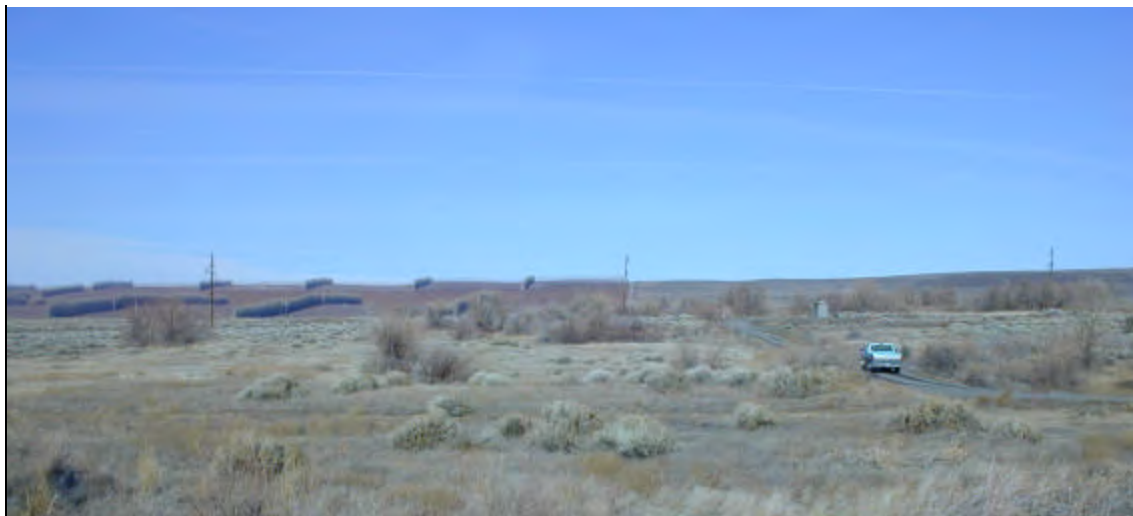
Photo 3.9-16. View of area near Vantage Substation
