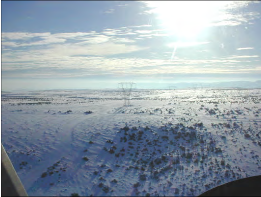
Photo 3.9-6. Aerial view of Schultz-Vantage Middle Canyon approaching the Columbia River
