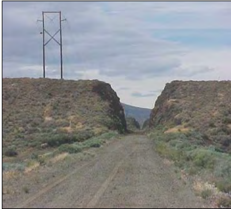
Photo 4.9-1. John Wayne Trail along Segment B SOUTH
