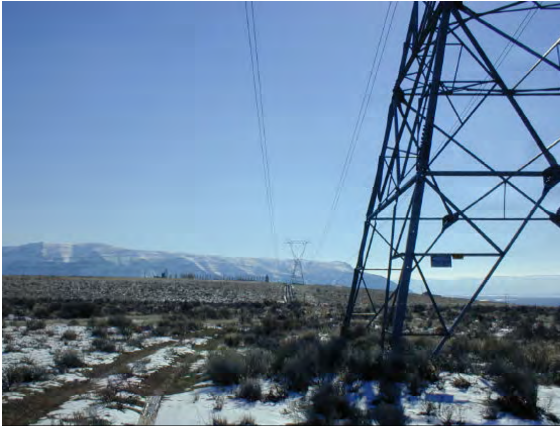
Photo 3.9-10. View of Vantage-Hanford transmission line from Vantage Substation looking south towards the Saddle Mountains
