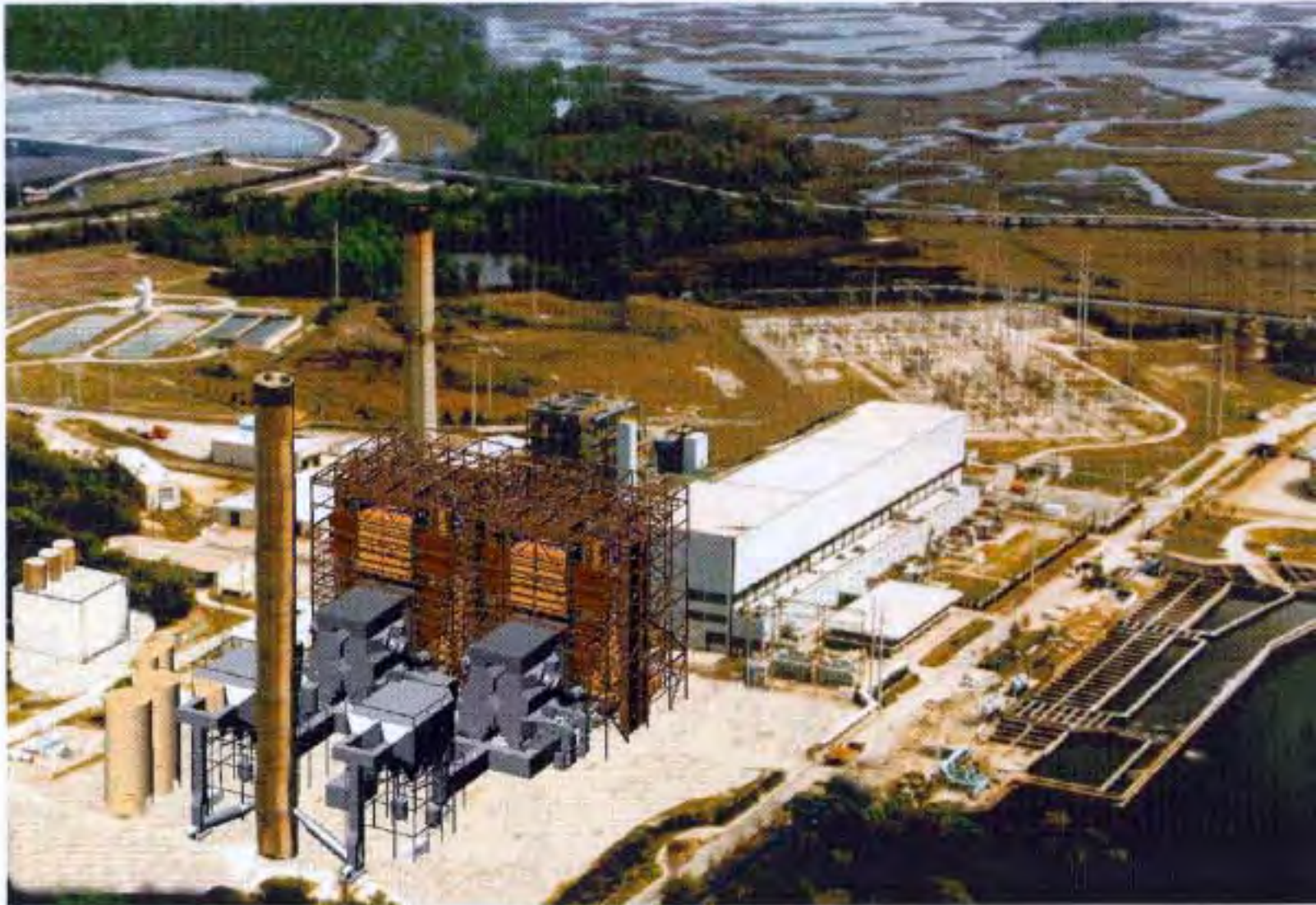
Figure 2.1.6. A computerized drawing of the proposed facilities superimposed on a photograph of the existing Northside Generating Station with the existing Unit 1 combustor and stack removed (view is to the northeast).
