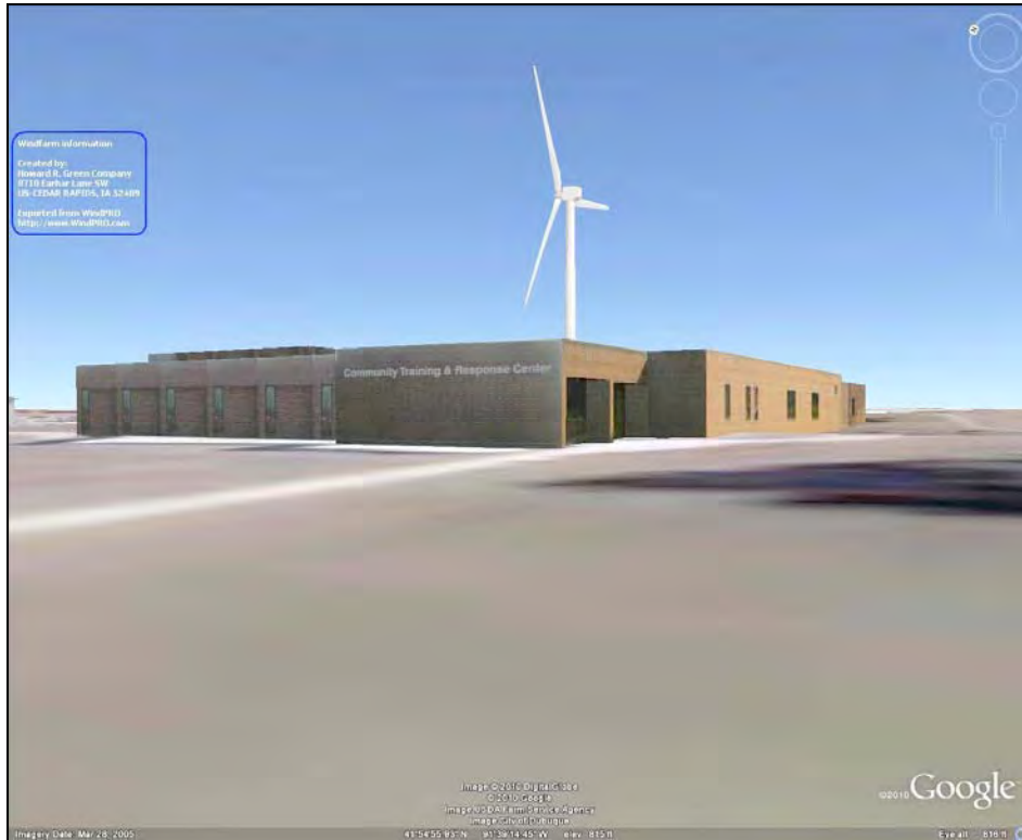
Community Training and Response Center. The nearest classroom building to the turbine.
