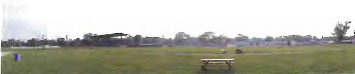
Location of Turbine, with Grandstands in Background
