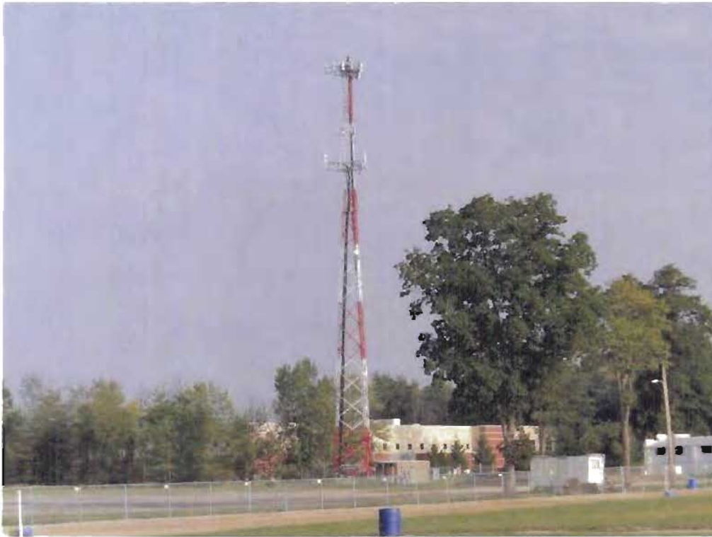
Communication Tower at Fairground, near the Turbine Site
