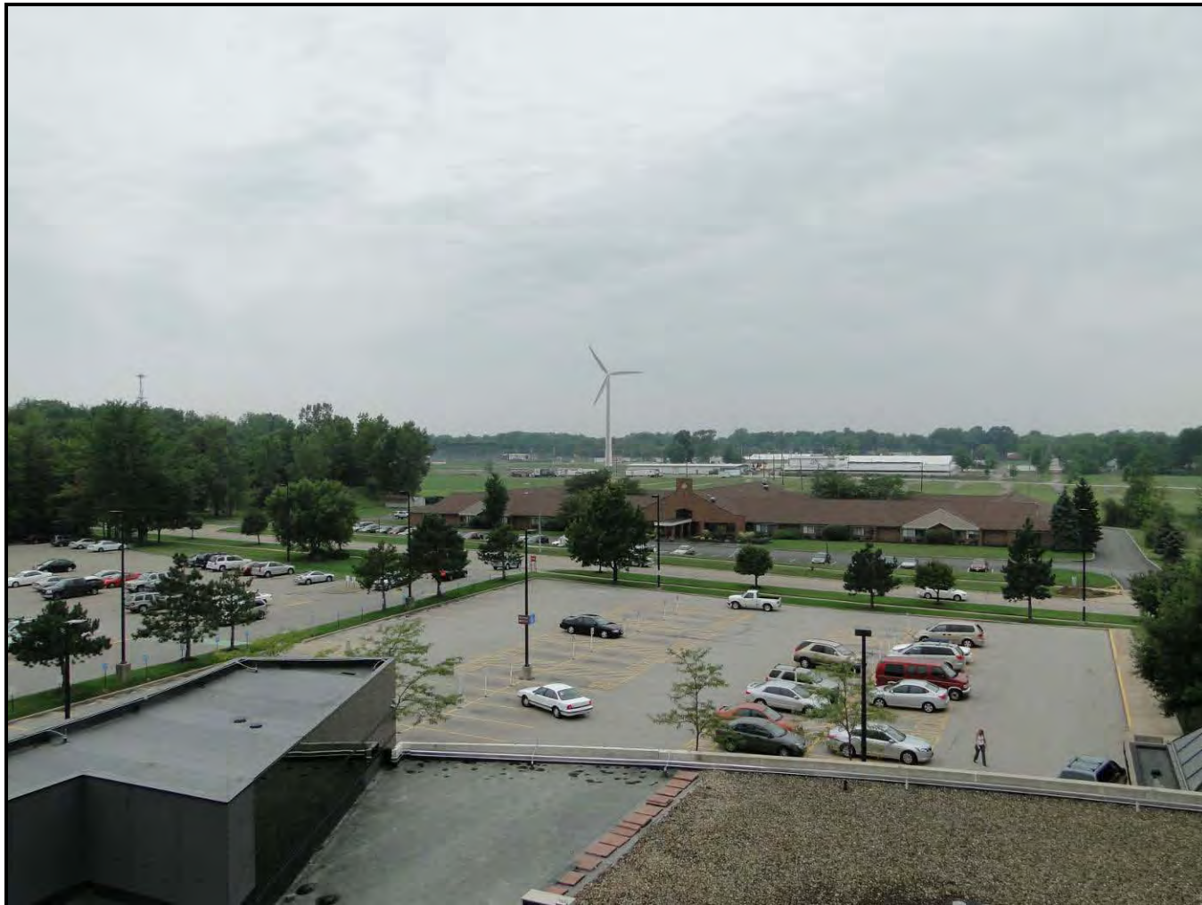
Southwest General Hospital Parking Garage Image taken from top of Parking Garage (49' off of Ground)
