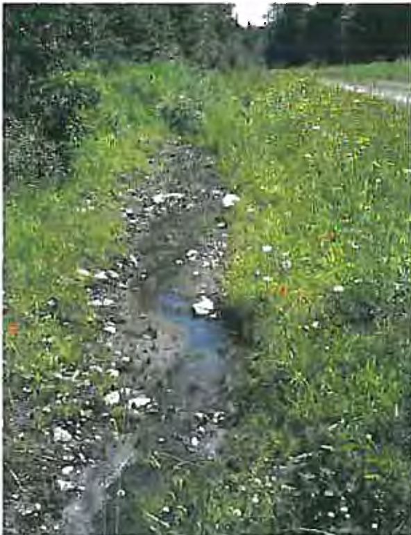
Photo 58-9A: Impact 58-9 Looking South
