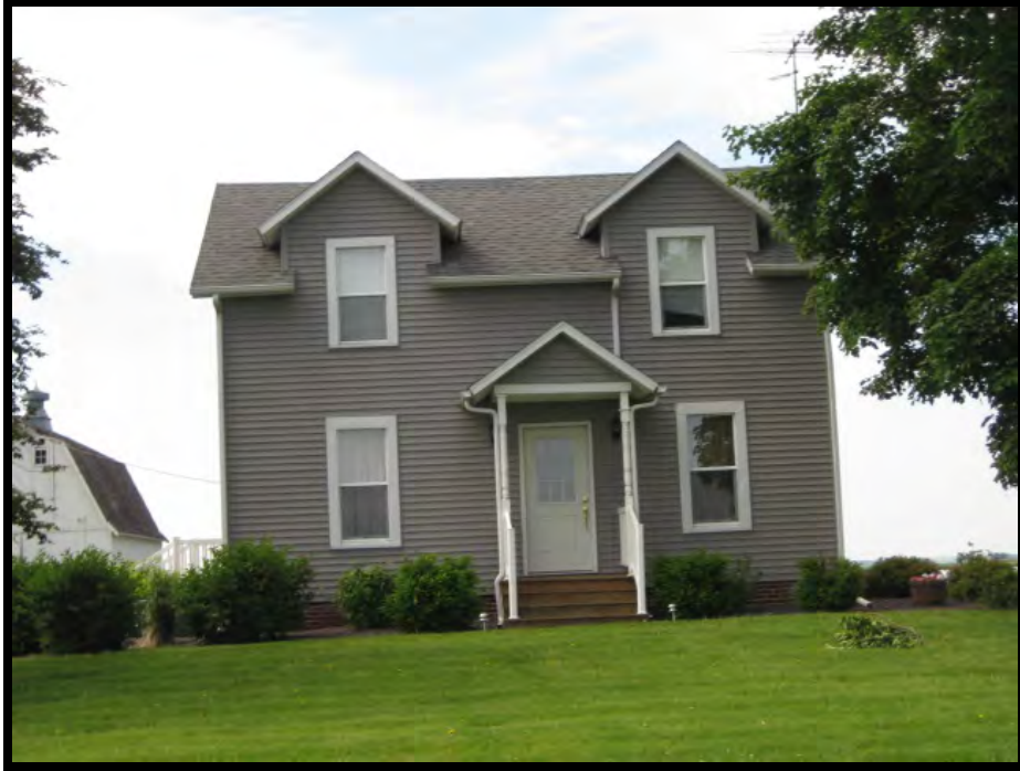
Photo 11 – Modified Resource M3, north elevation.
