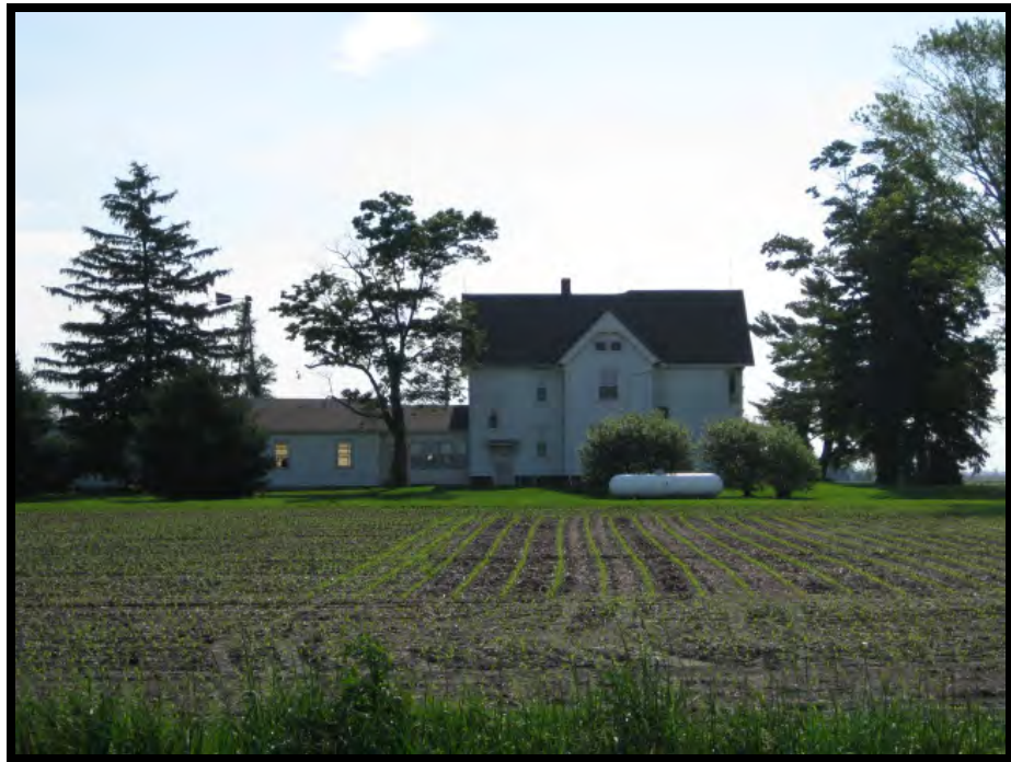
Photo 2 – Architectural Resource A1, west elevation.
