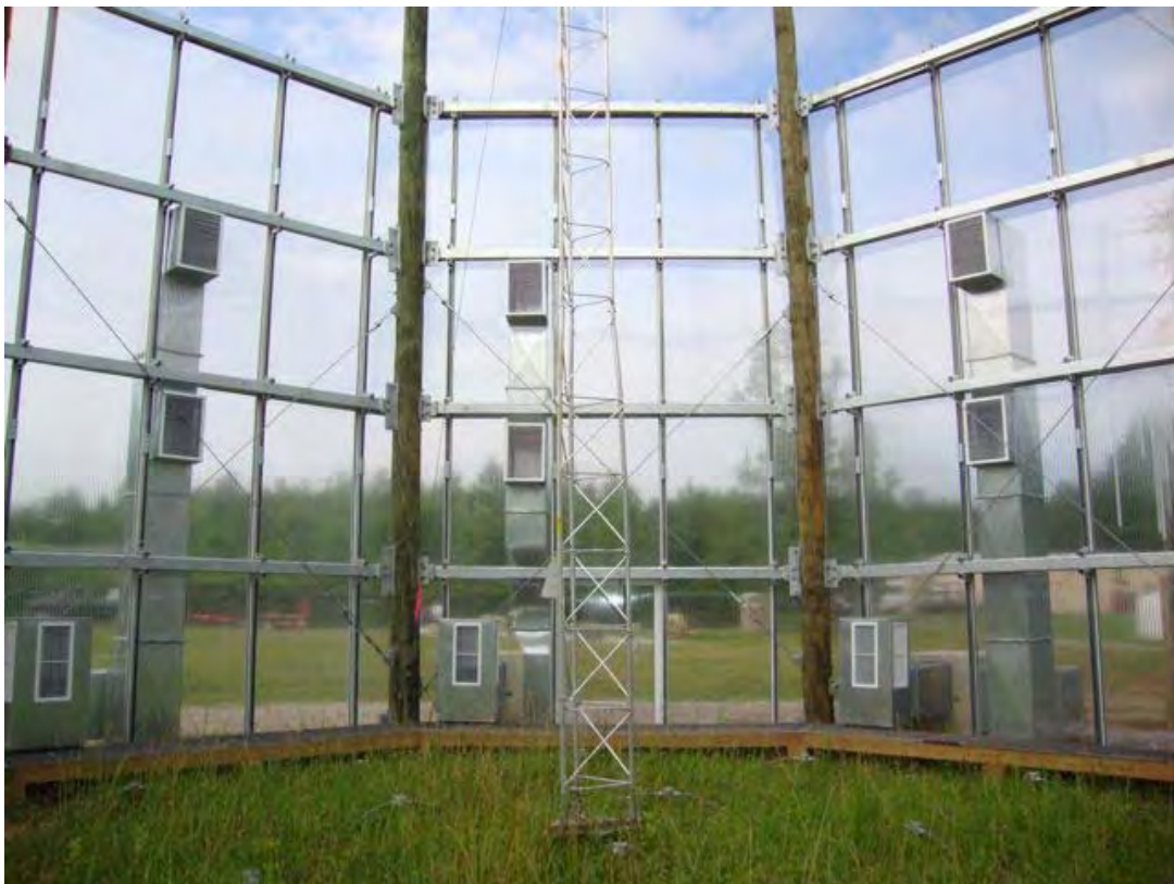
Fig. 2.5. Exterior and interior views of the prototype 12-m (39-ft) diameter warming enclosure constructed in Oak Ridge, Tennessee.
