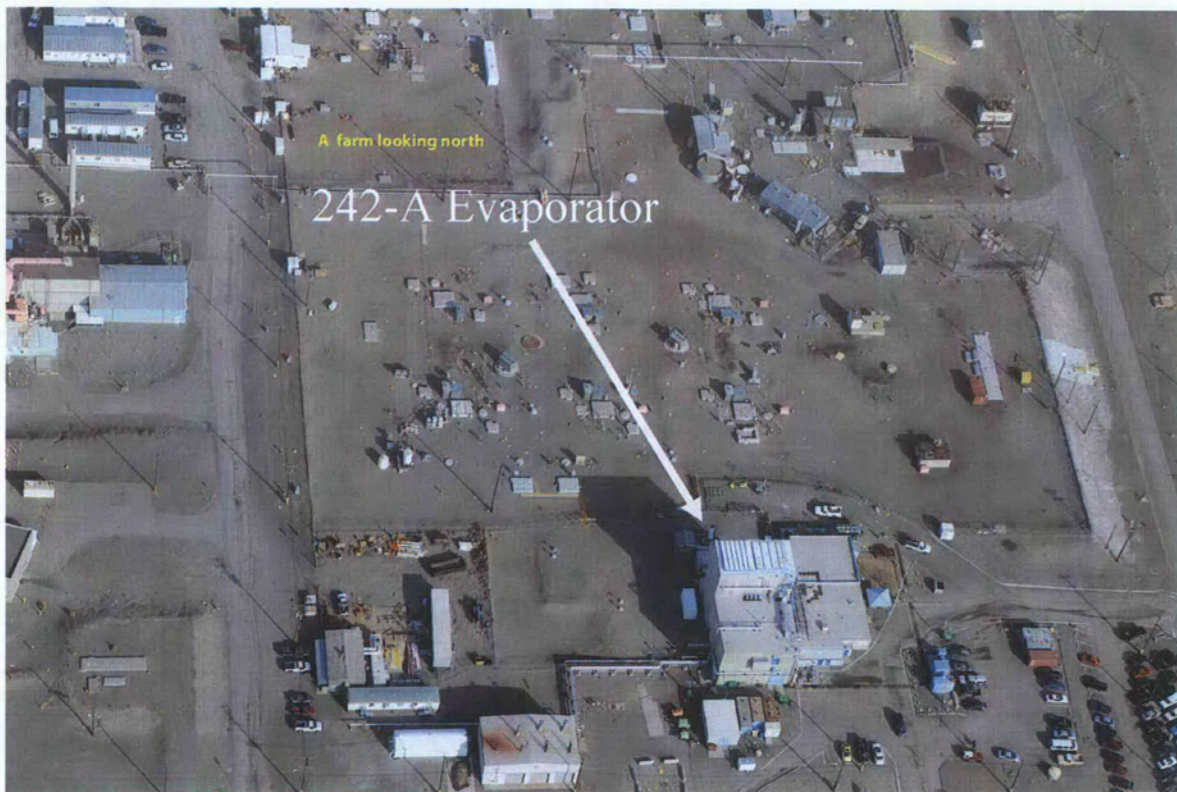
Figure 5. 242-A Evaporator Aerial View.
