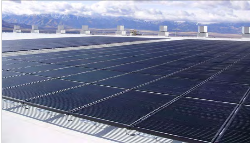
Figure 2-2 Solyndra Rooftop Installation
