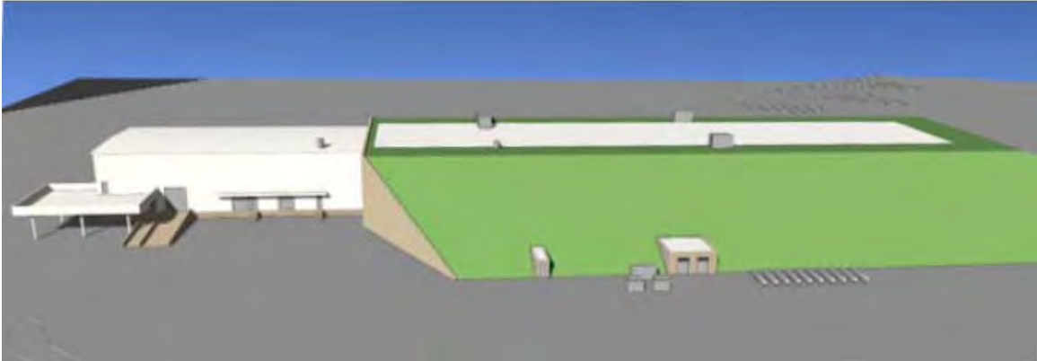
Figure 3.9: A perspective view of the proposed NOvA Far Detector building looking east. The bermed area (green) is composed of granite spoils from the excavation. The detector area would be on the right hand side with a module assembly area to its left. A loading dock service area is located to the left of the Assembly Area with recessed and drive-in truck bays. A scintillator tanker handling area is shown on the far left with adjacent bays for four tanker trucks.
