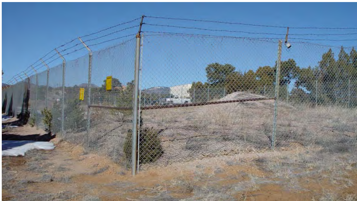
Figure 4. Material Disposal Area H at TA-54. (The mound of soil in the right forefront of the photo is clean fill remaining after the excavation of the last shaft.)
