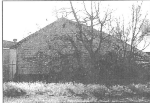
Small Arms/Ammunition Storage (Building 33)
