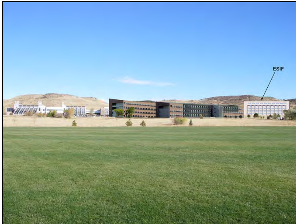
Figure 3-4. ESIF Option A – View From South (including the Research Support Facility currently under construction)
