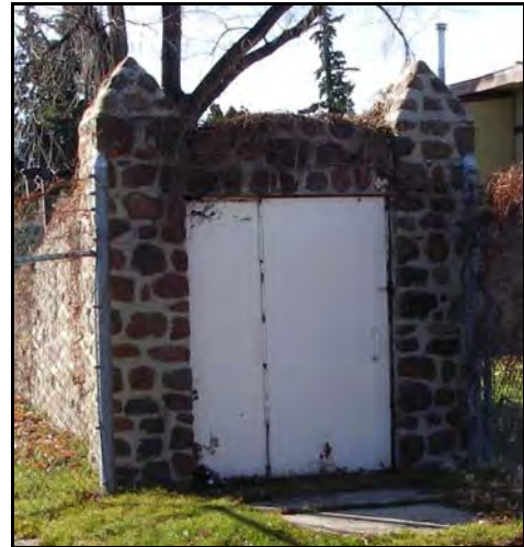
Pedestrian Underpass (Structure 50)
