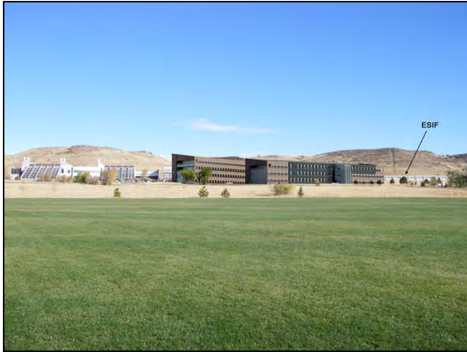
Figure 3-5. ESIF Option B – View From South (including the Research Support Facility currently under construction)
