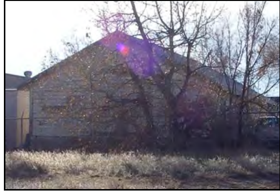
Small Arms/Ammunition Storage (Building 33)
