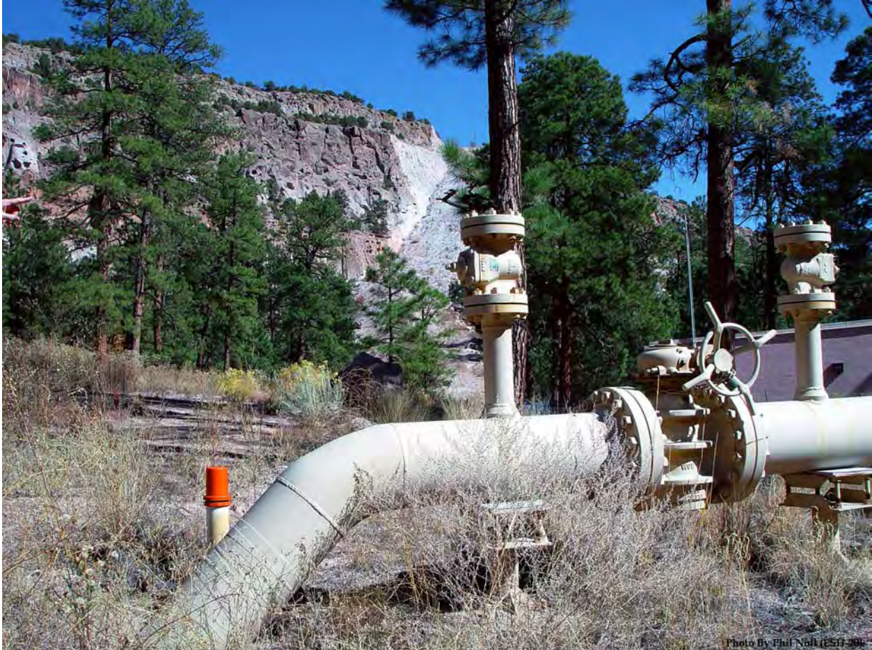
Figure 3. Existing aboveground 12-in. (30-cm) PNM gas mainline valve in Los Alamos Canyon.
