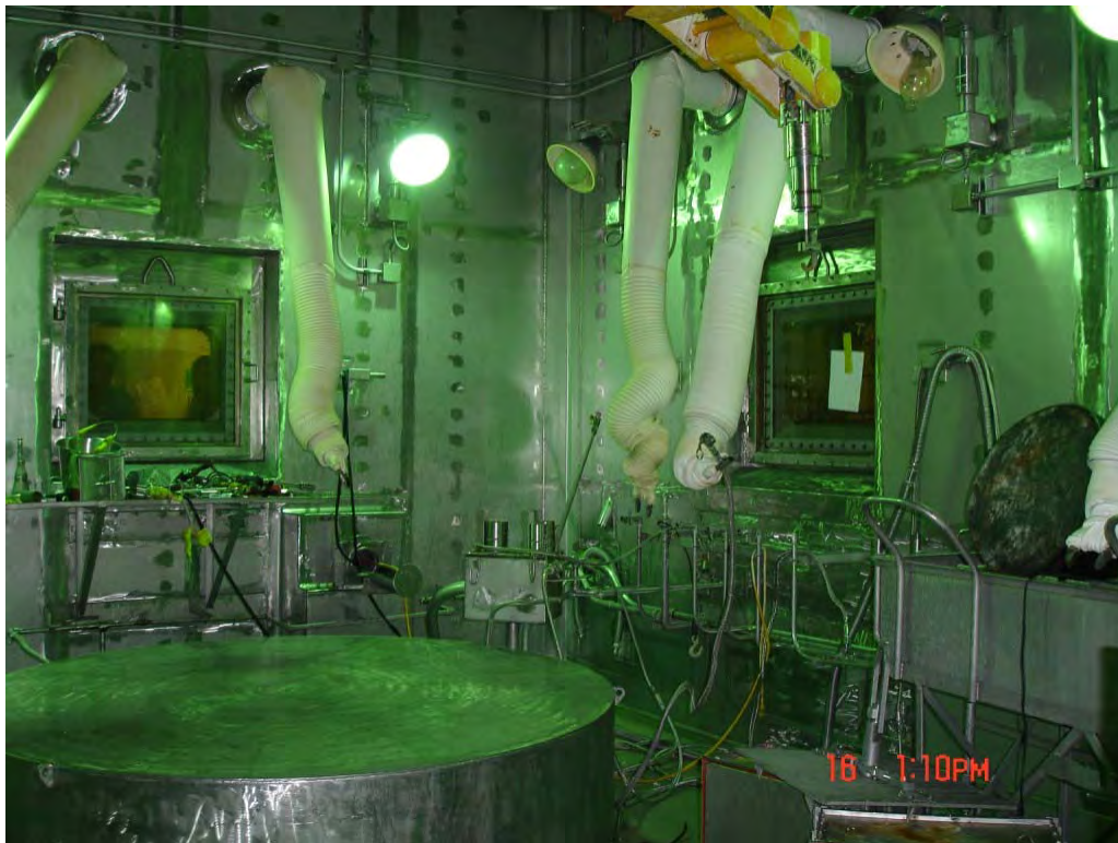
Figure 10. New Waste Calcining Facility Cell 308 interior.
