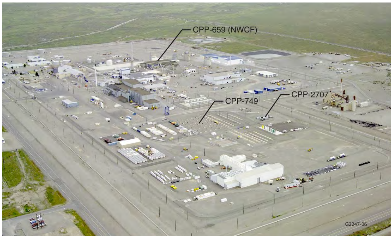
Figure 9. Location of CPP-659, CPP-749, and CPP-2707 at the Idaho Nuclear Technology and Engineering Center.
