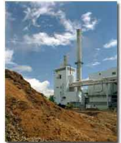
Biomass Power Plant - Photo credit: U.S. Department of Energy, Energy Efficiency & Renewable Energy Network (EREN)
