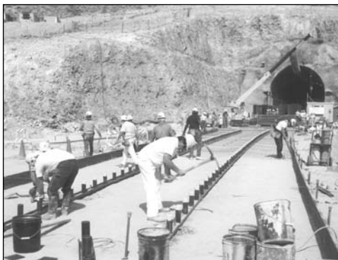
Yucca Mountain construction activities
