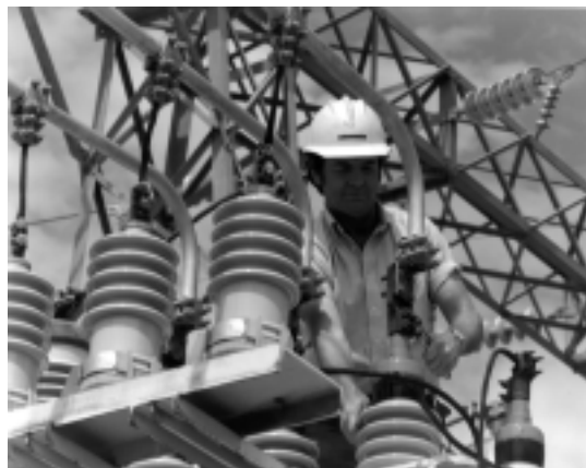
Southwestern Power Administration's Poplar Bluff, Missouri, switchyard.
