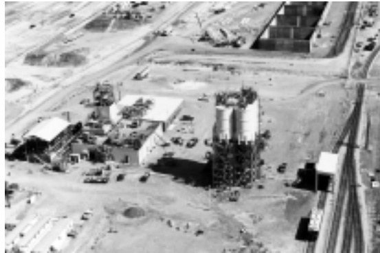
Saltstones low-level waste solidification and disposal at Savannah River Site.
