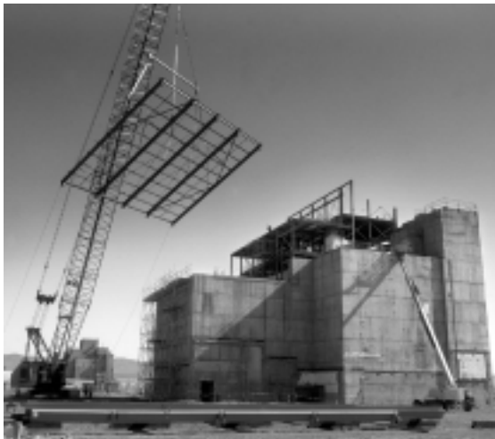
Hanford Site—A new roof structure is being constructed to safely enclose the 100-DR Reactor Core.
