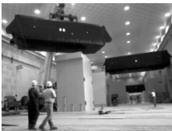
Installation of NIF Spatial Filter End Vessels in Laser Bay 2 at Lawrence Livermore National Laboratory.
