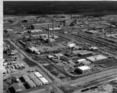
Aerial view of tritium facilities at Savannah River
