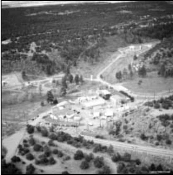
Technical Area-18, Los Alamos National Laboratory
