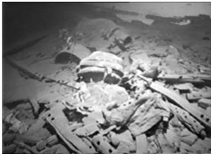
Sludge and debris in the K East Basin at the Hanford Site
