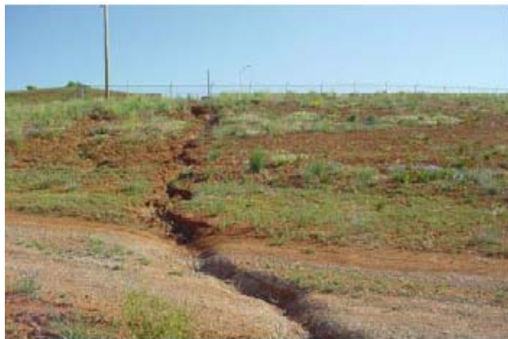
Erosion at the Monticello Mill Site
