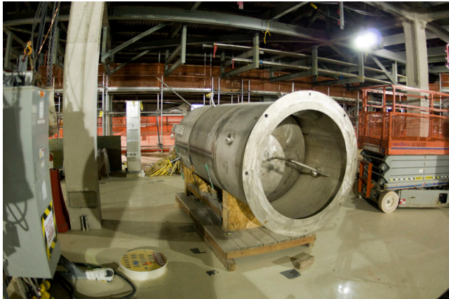
Equipment installation activities
