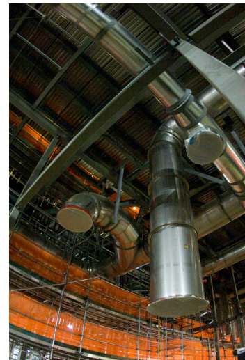
Overhead piping installations
