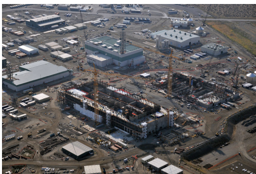
Aerial view of the WTP primary facilities
