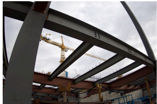
Structural steel at the High Level Waste facility
