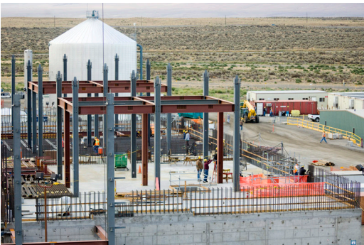
Structural steel installed on High Level Waste facility
