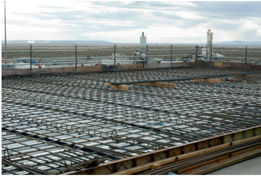
Installed rebar and decking awaiting concrete on the Low Activity Waste facility export bay roof
