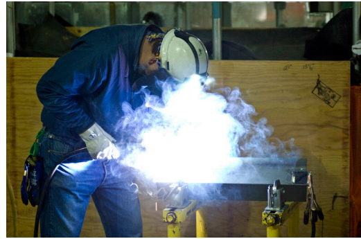
Worker welds a piece of steel beam in the Low Activity Waste facility hot cell area
