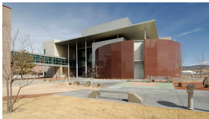
MicroFab Facility at SNL
