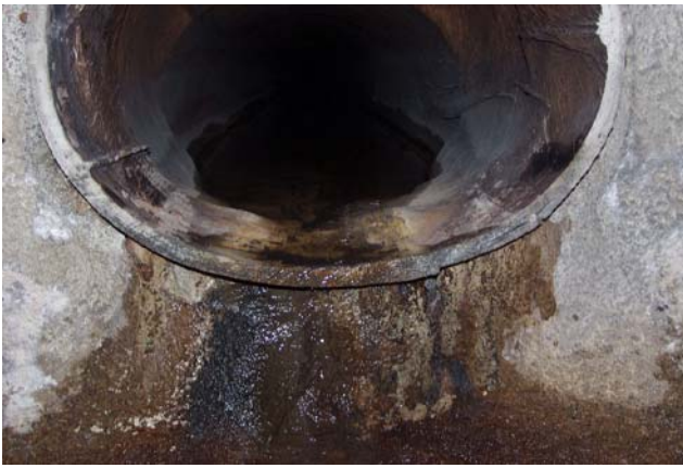
Lined Lateral Pipe
