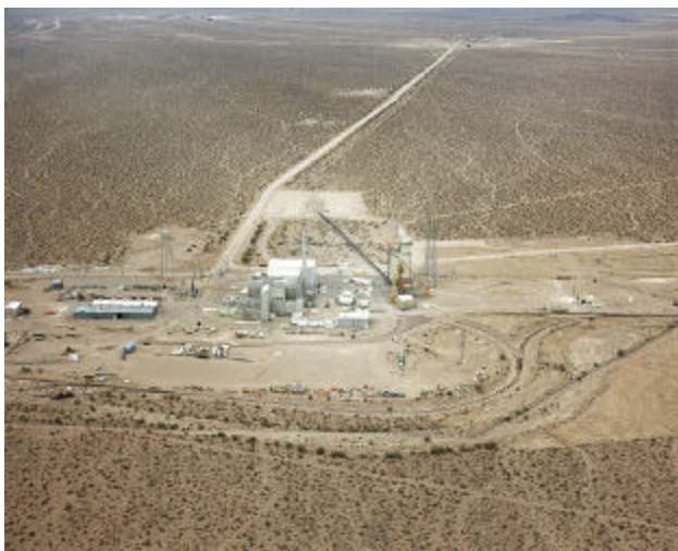
Reactor Maintenance Assembly and Dissassembly Facility
