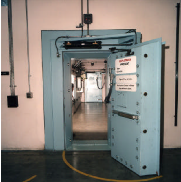
Device Assembly Facility Explosives Handling Room
