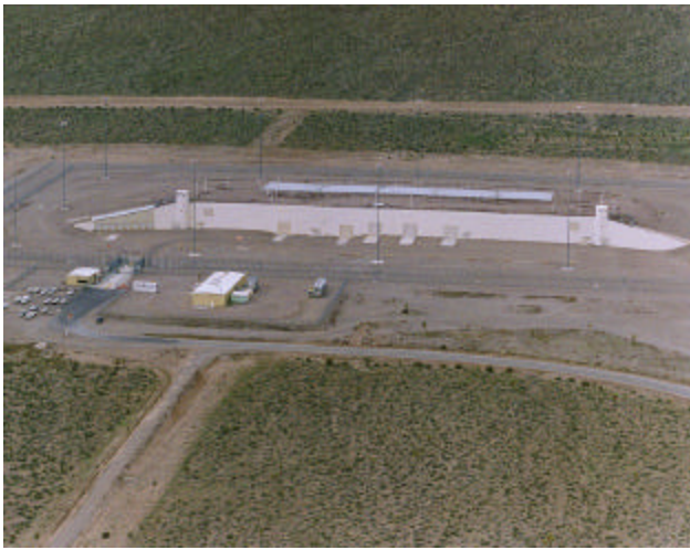
Exterior View of DAF
