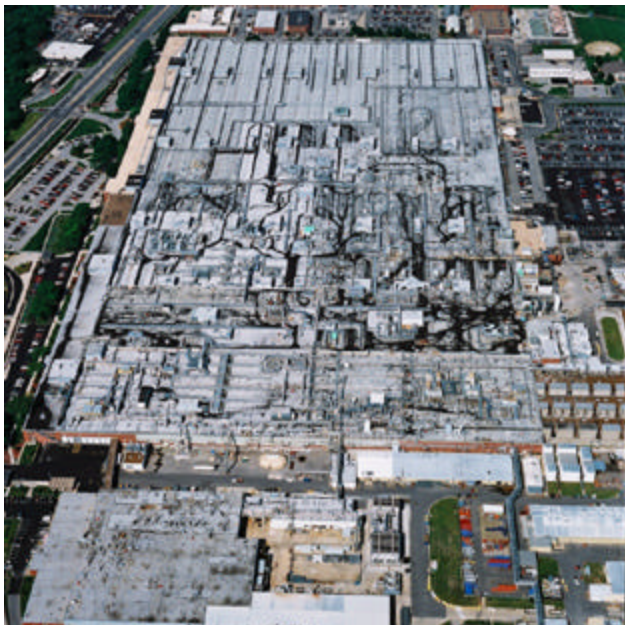
Aerial of Kansas City Plant Roof
