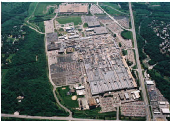
Aerial View of Kansas City Plant
