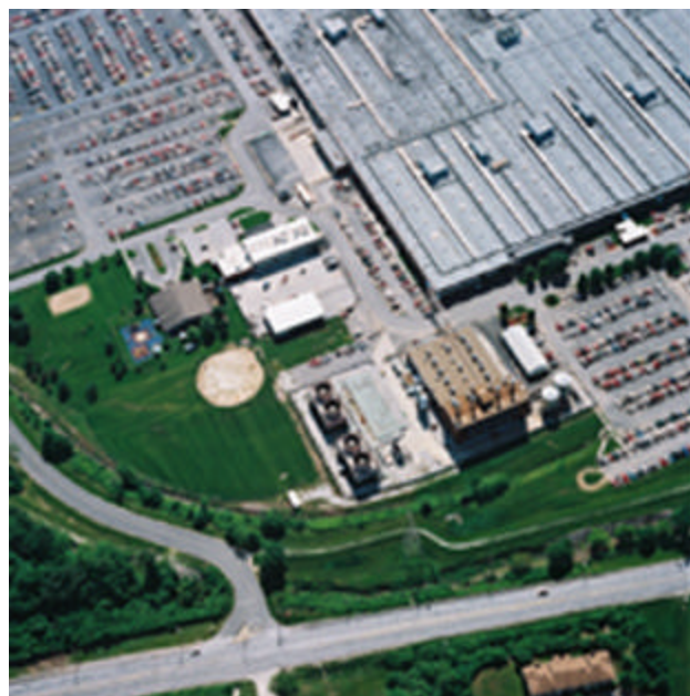
Aerial View of West Boiler House
