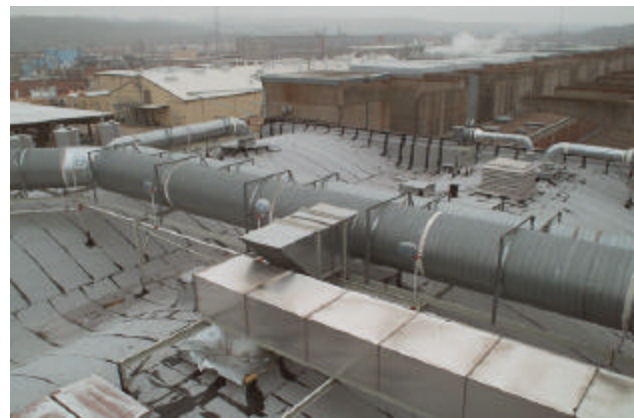
Ventilation Systems on Roof Area
