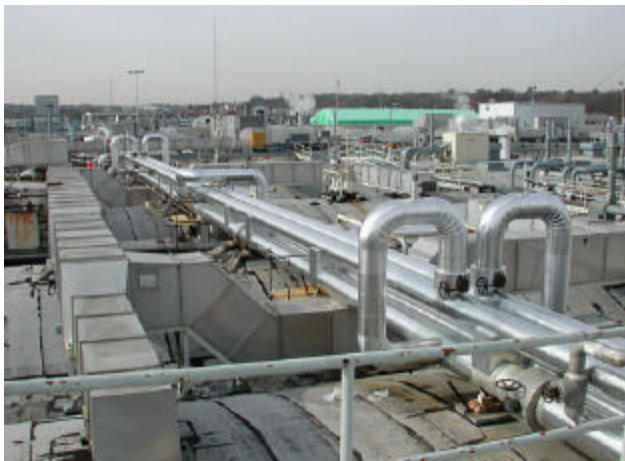
Kansas City Plant Roof Area
