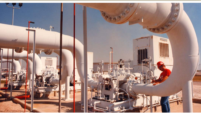
With a capacity of 727-million-barrels, the U.S. Strategic Petroleum Reserve is the largest stockpile of government-owned emergency crude oil in the world.
