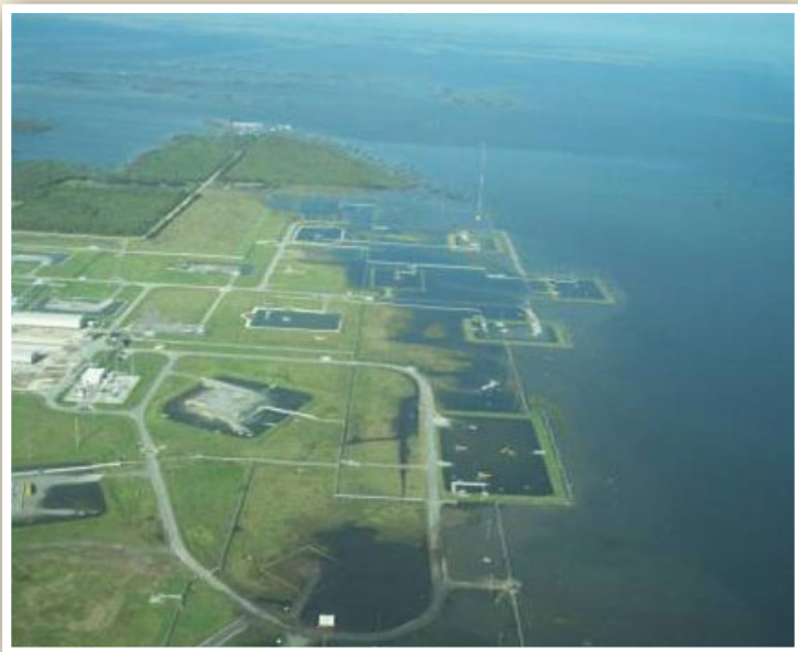
The flooded surface of Cavern Six at the West Hackberry, La., site after a hurricane.
