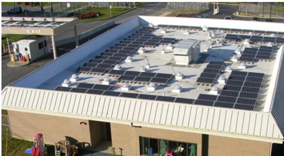
Photovoltaic arrays and solar light tubes on the NETL-Morgantown Daycare Facility.
