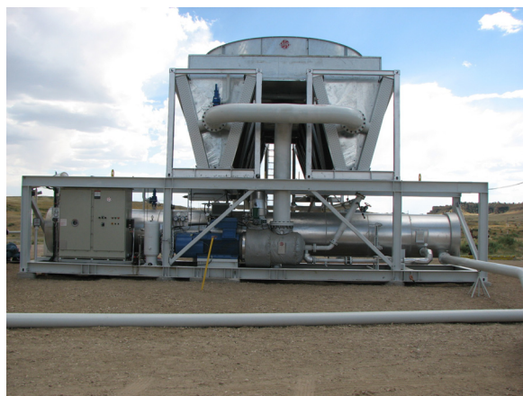
A geothermal electric power generator at RMOTC.
