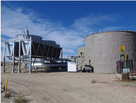
ORMAT geothermal facility at RMOTC.
