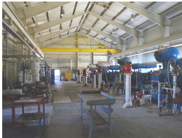
RMOTC inactive low-temperature separation gas plant after purge and drain.
