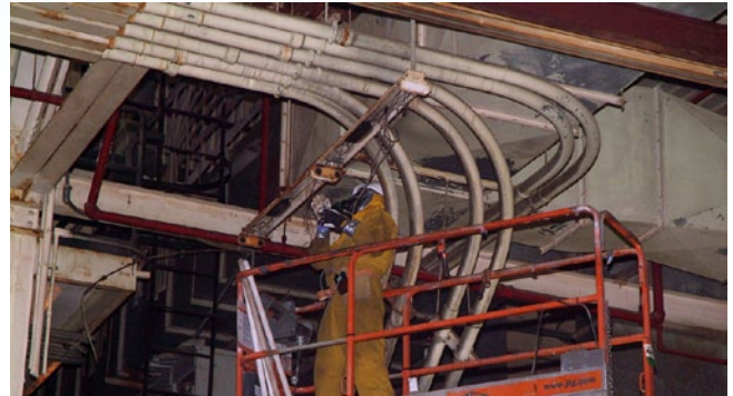
A Recovery Act worker removes a light fixture in the Metals Plant to prepare the facility for demolition.
