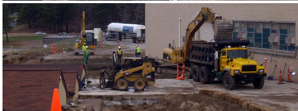
Top: Recovery Act workers demolish the Building 802 Fan House.
