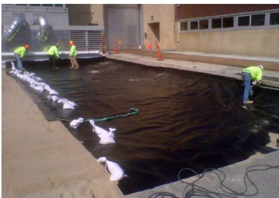
Above photos: Recovery Act workers install a portion of the impermeable cap at the Brookhaven Graphite Research Reactor.
