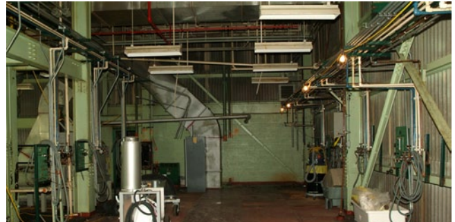
Uranium hexafluoride valve test cabinets (middle above), line a section of the fifth floor of the C-340 Metals Plant before cleanup. Directly above, the cabinetry is gone.
