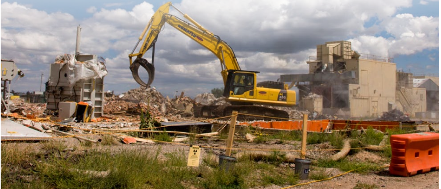
Multiple Recovery Act projects are ahead of schedule at LANL, including the demolition of 24 buildings at Technical Area 21.
