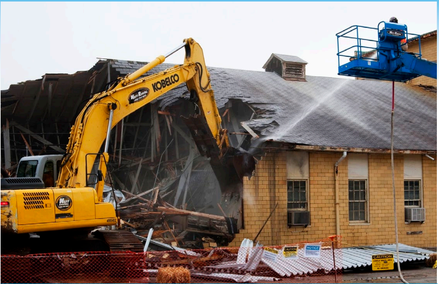
Workers demolish a building on Y-12 National Security Complex's Engineering Row.
