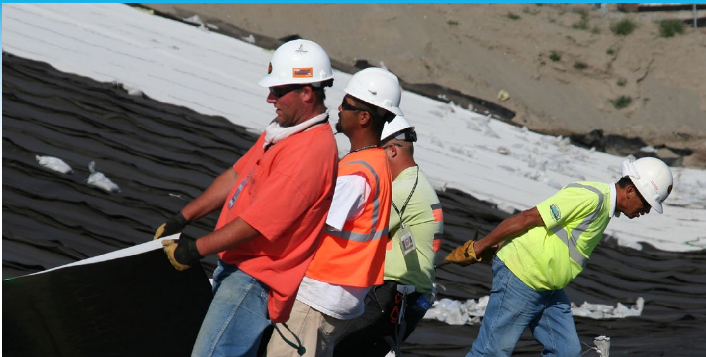
Workers install a liner in a disposal facility at the Hanford Site to protect the groundwater from contamination. The Recovery Act is funding the expansion of the facility to increase its capacity by 50 percent, enough to hold more than 16 million tons of low-level waste from environmental cleanup activities at the Hanford Site.
