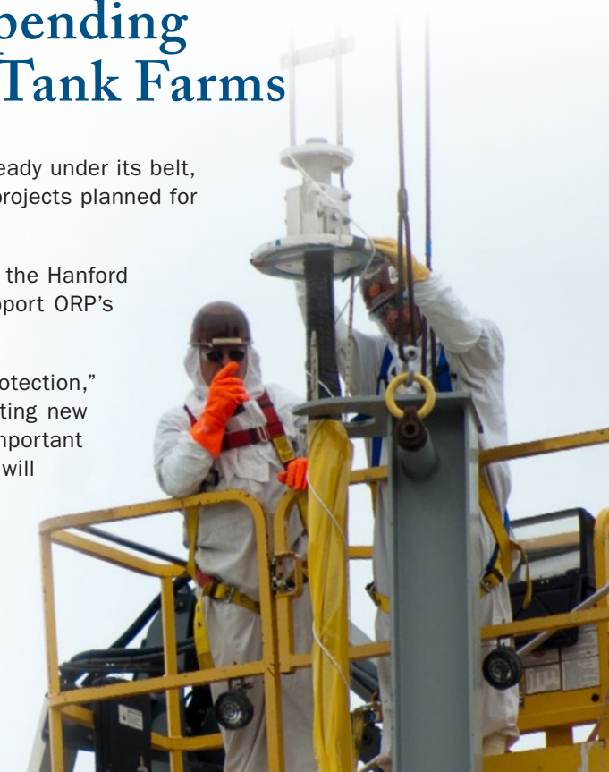
Workers install a liner in a disposal facility at the Hanford Site to protect the groundwater from contamination.
