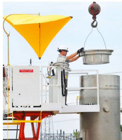
Workers load drums of transuranic waste into a custom-designed container to be transported to the Waste Isolation Pilot Plant in New Mexico for disposal.
