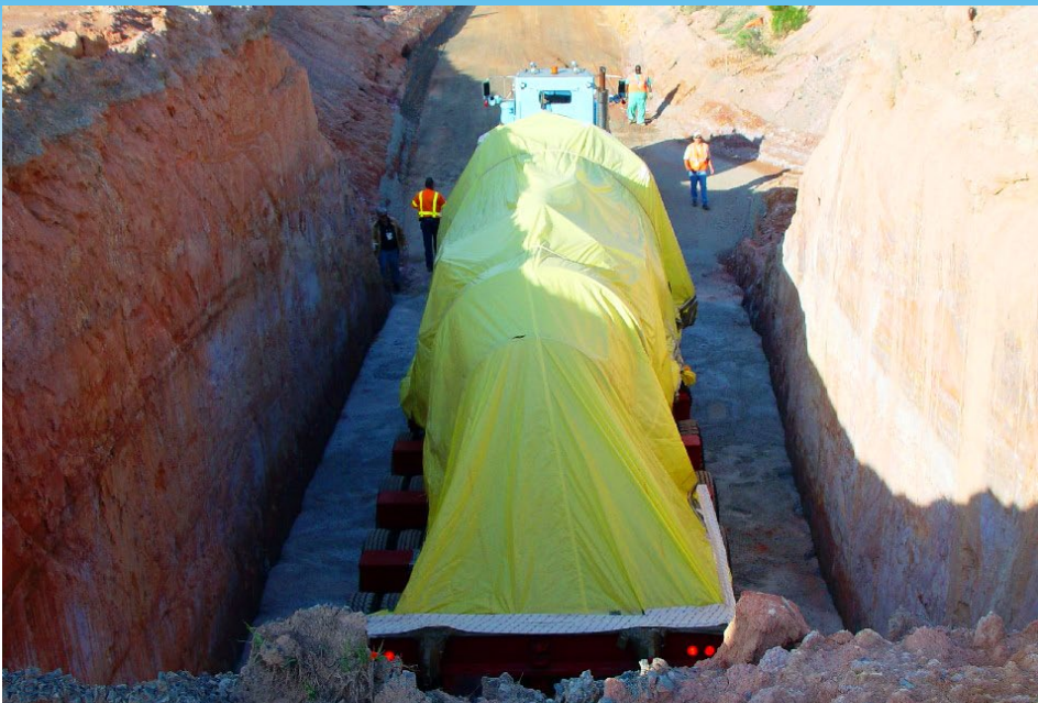
Recovery Act workers removed the Heavy Water Components Test Reactor vessel, shown here, and permanently disposed it onsite.
