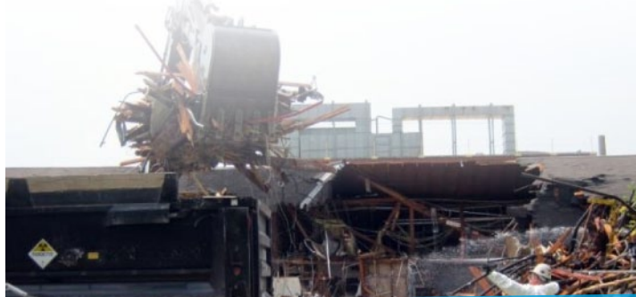
Workers demolish Building 3550 in the Oak Ridge National Laboratory's central campus. It was the twelfth building to be decontaminated and demolished in the 34-facility decontamination and demolition project.
