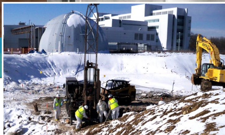
A drill-rig crew takes soil sample bores for analysis as part of decontamination and demolition of Argonne's Building 330, the former site of the historic Chicago Pile-5, the fifth and final member of the Chicago Pile family of pioneering research reactors.
