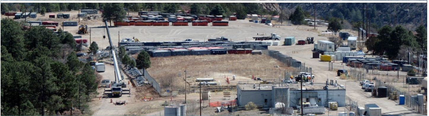
These photos show the DP East area of Los Alamos National Laboratory's Technical Area 21 before the demolition of 10 buildings, above, and after demolition, below.
