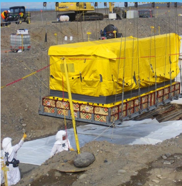
Top Photo: Workers lift a large box of transuranic waste covered in protective plastic and a shoring base from an underground storage trench.
