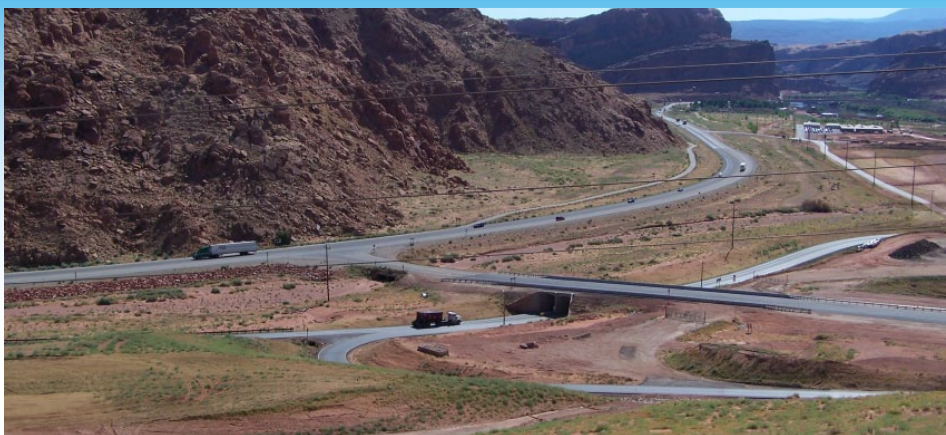
A truck carrying a container full of tailings exits the underpass (center of photo) and heads up the paved haul road to the rail load out area.
