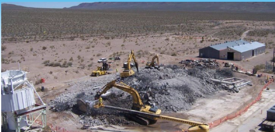
Recovery Act crews remove demolition debris at the Reactor Maintenance, Assembly, and Disassembly Facility.
