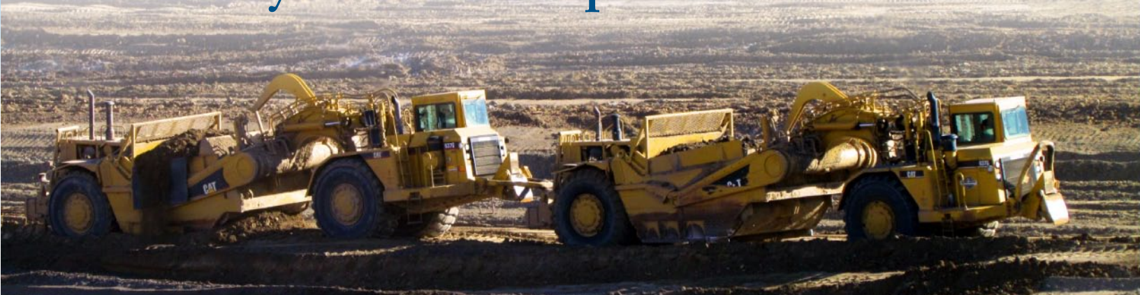
Two scrapers work together to excavate Mancos Shale at the Crescent Junction site to create the second portion of a disposal cell for uranium mill tailings.
