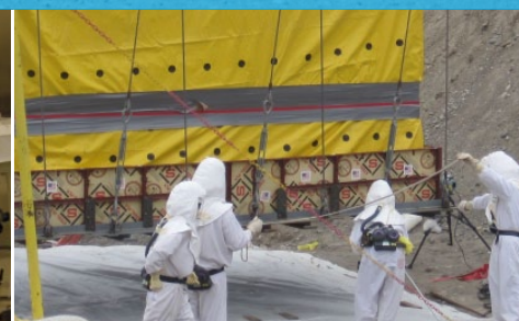
A box of transuranic waste is removed from an underground storage trench at the Hanford Site.
