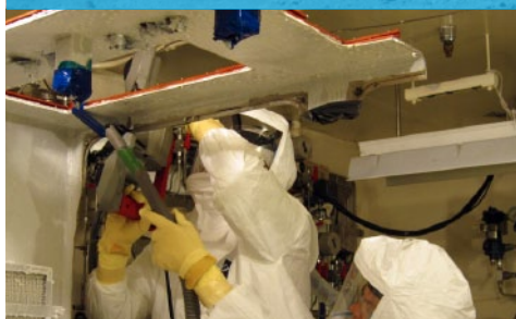
Workers cut up a glovebox in the 209-E Criticality Mass Laboratory, one of the last buildings being prepared for demolition on Hanford's Central Plateau.
