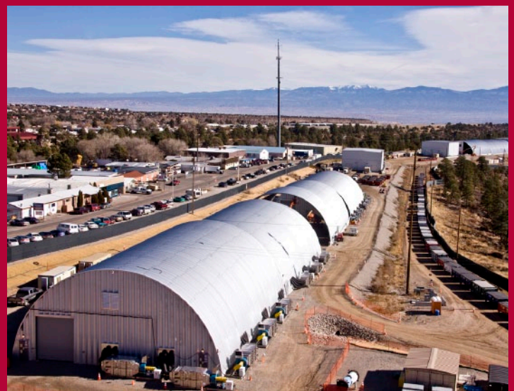
The excavation of MDA-B was done inside sturdy metal buildings.
