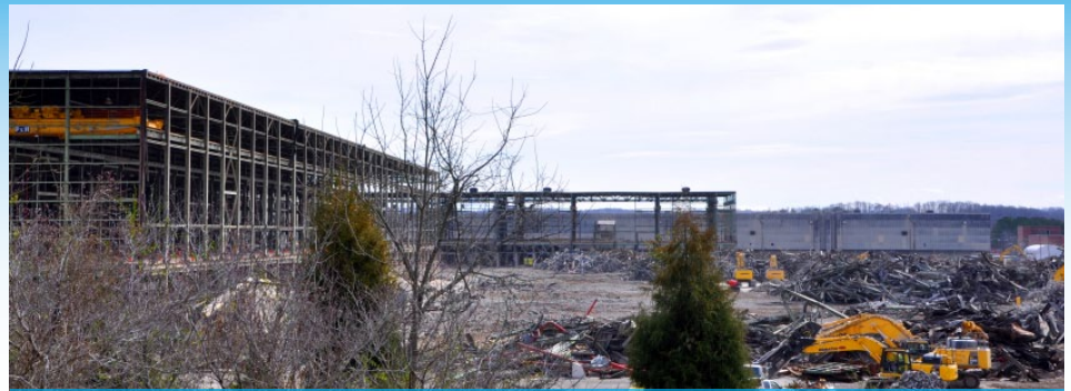
Earlier this year at the East Tennessee Technology Park, workers demolished the Building K-33, which measured 1.4 million square feet.
