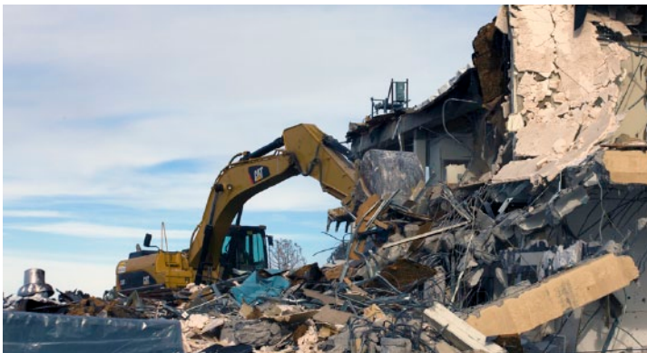
The demolition of 24 buildings at Technical Area 21 at Los Alamos National Laboratory was completed six months ahead of schedule.
