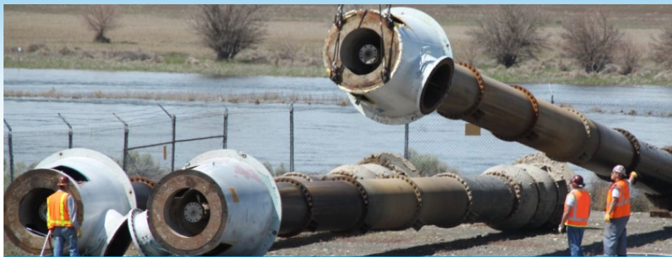
Pump structures from the 181-KE River Pump House are lowered via crane after removal from the riverside structure. The structures will be cut up and disposed at Hanford's Environmental Restoration Disposal Facility.
