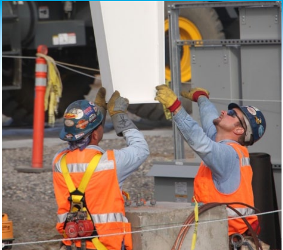
At the Hanford Site in Washington state, construction of the 200 West Groundwater Treatment Facility is on track to be completed by September 2011.
