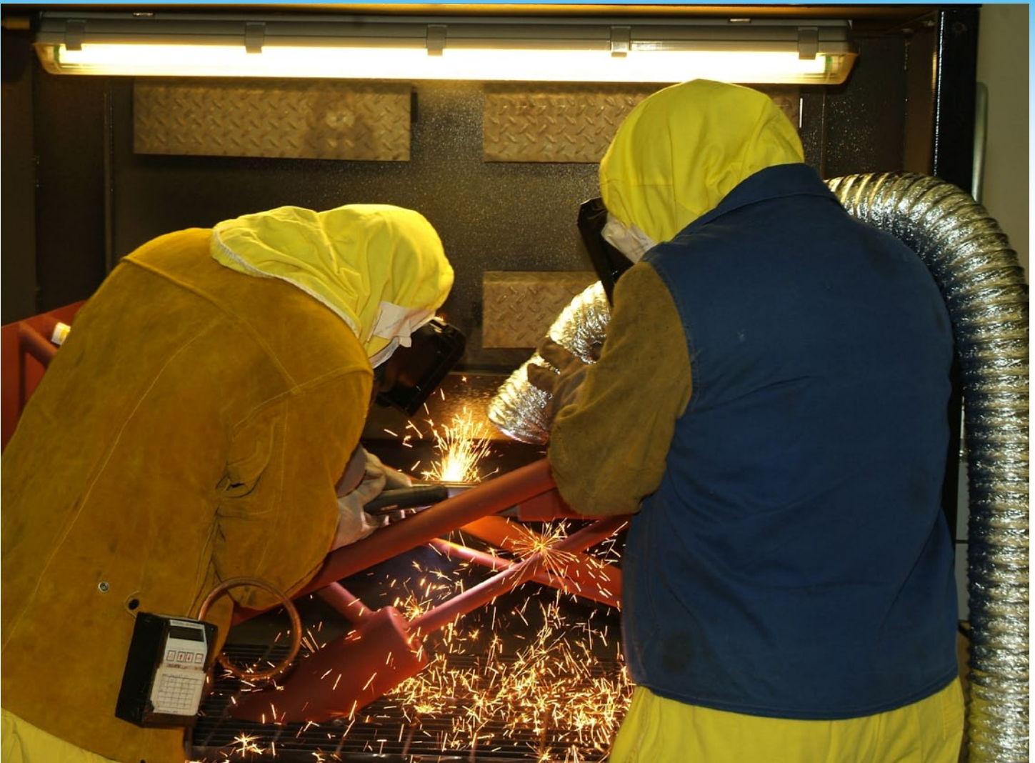
Maintenance mechanics train with plasma arc-cutting equipment prior to removing miles of piping from old buildings at the Paducah Site.
