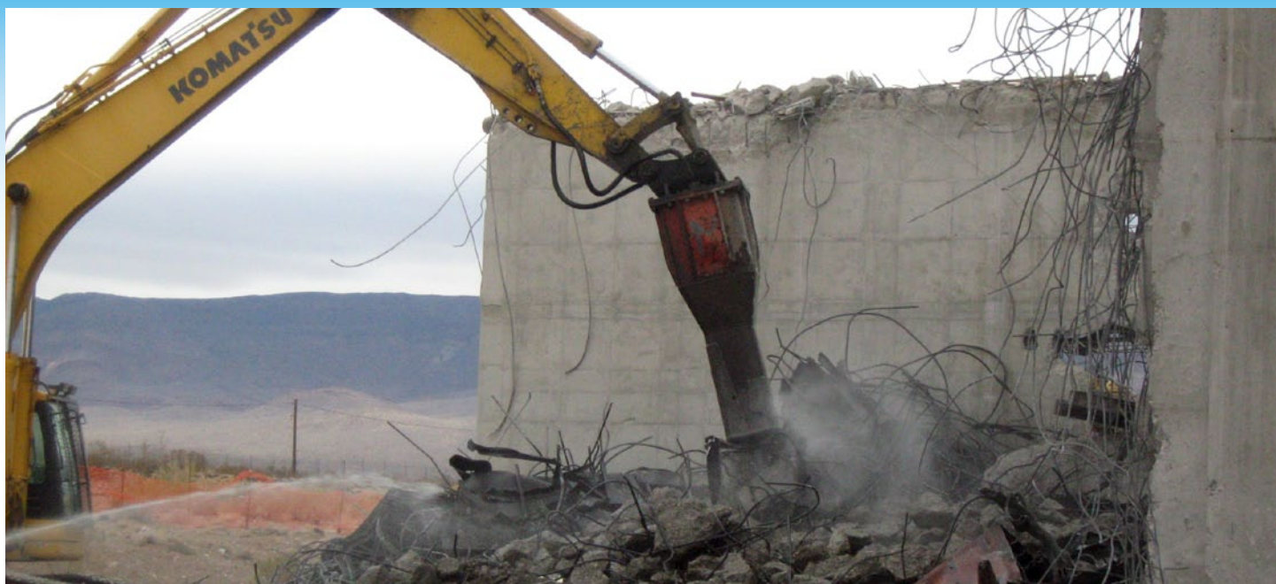
The Nevada Site Office identified the demolition of the Reactor Maintenance, Assembly, and Disassembly Facility as a top Recovery Act accomplishment at the Nevada National Security Site in 2010.
