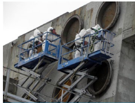
Recovery Act workers close ducts as part of ongoing efforts to decommission the P Reactor, which formerly supported the production of nuclear materials.
