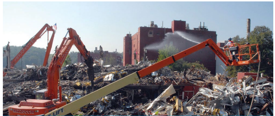
Workers demolish a facility at the Biology Complex at Y-12 National Security Complex, a 2010 accomplishment at Oak Ridge. The Recovery Act funded the demolition of four facilities at the Biology Complex, reducing the site’s footprint by 135,000 square feet.
