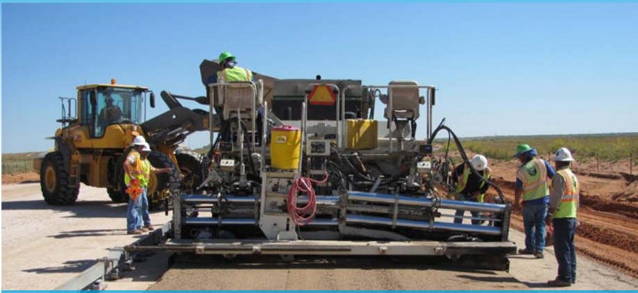
The reconstruction of a portion of the South Access Road was one of the Waste Isolation Pilot Plant's 2010 Recovery Act accomplishments.
