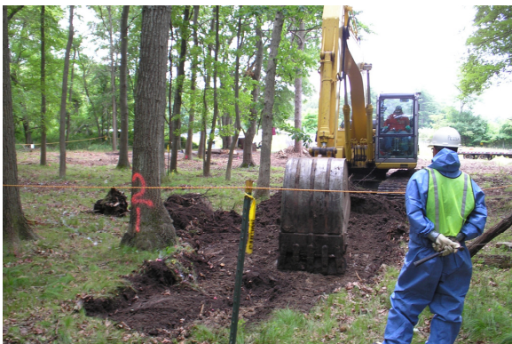
(Above) Soil Excavation and Waste Packaging in Progress
